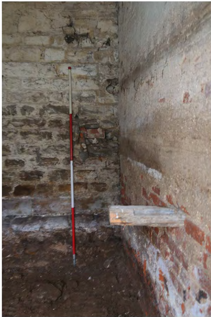
082_2000_2240-2103_trough W wall
