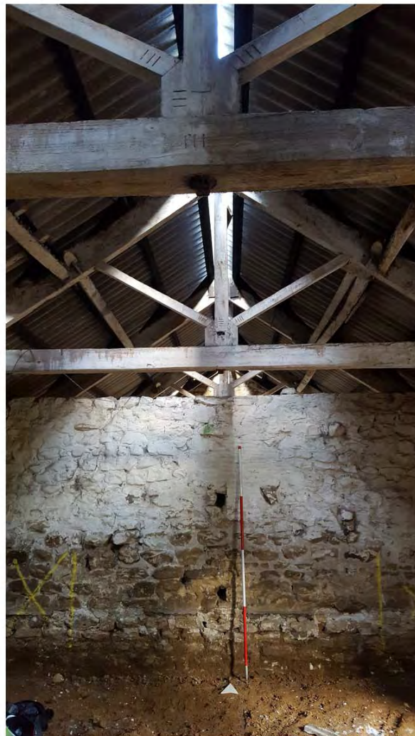
119-200_roof detail_carpenters marks III 200 both trusses and 204
