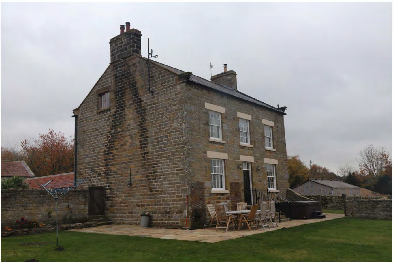
115_Gen_view of_house oblique lk NE
