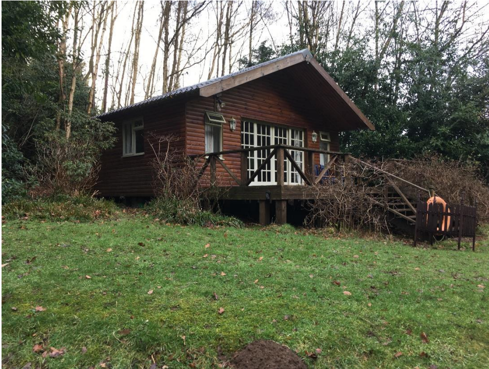
Fig 6. – height of the structure, steps to deck and void beneath
