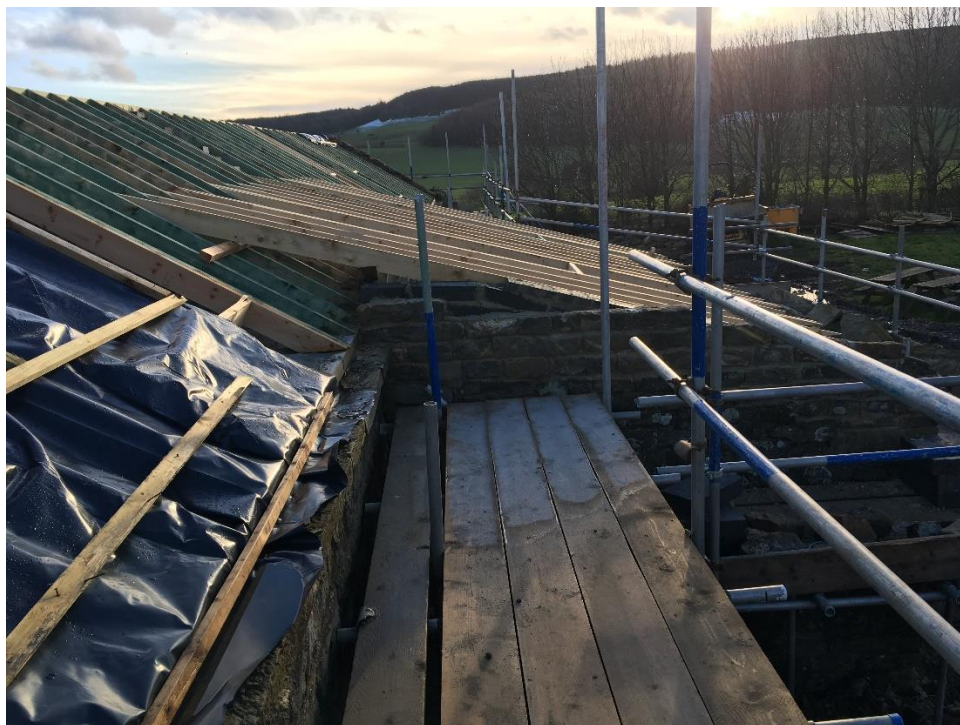
Photo 3 Lean-to roof over Kitchen/Dining, Mulberry Cottage
