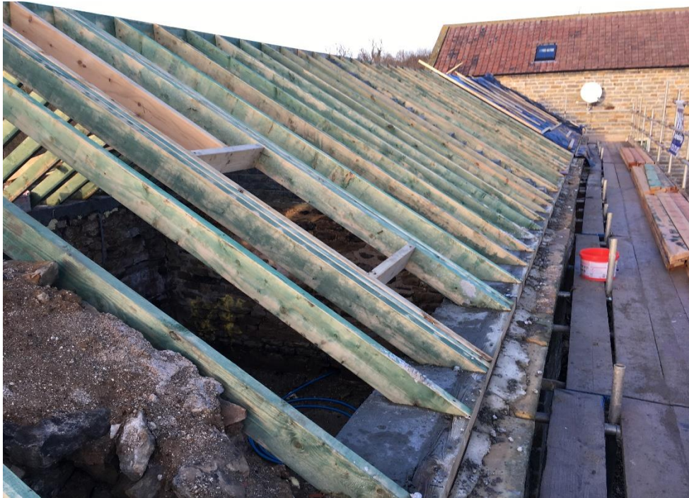
Photo 1 Roof over Bedroom 1, Hornbeam Cottage
