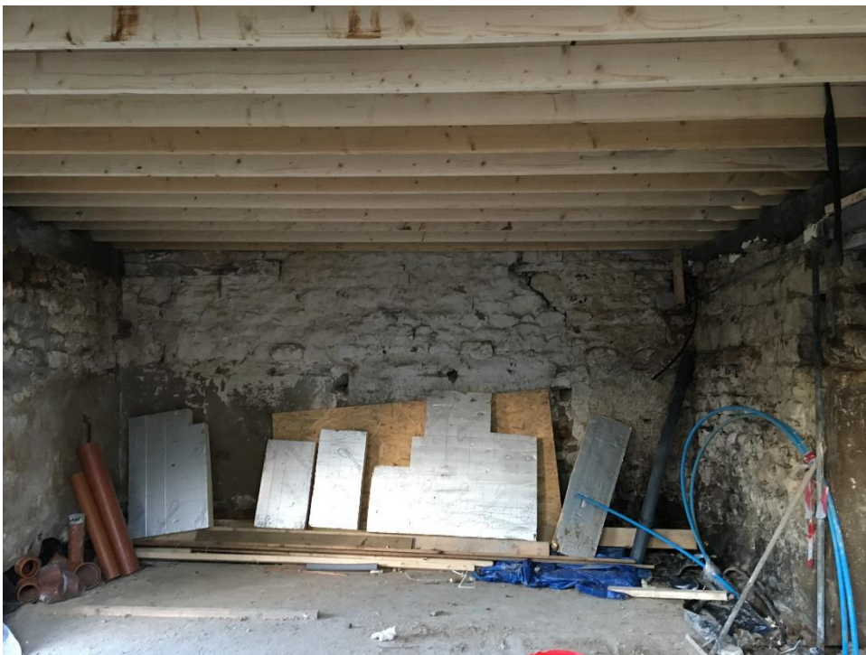
Photo 2 Roof/ceiling over Beds 1 and 2, Mulberry Cottage
