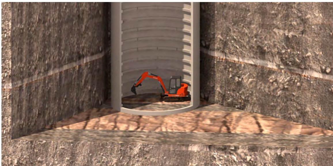
Mechanical Excavation Within the Shaft
