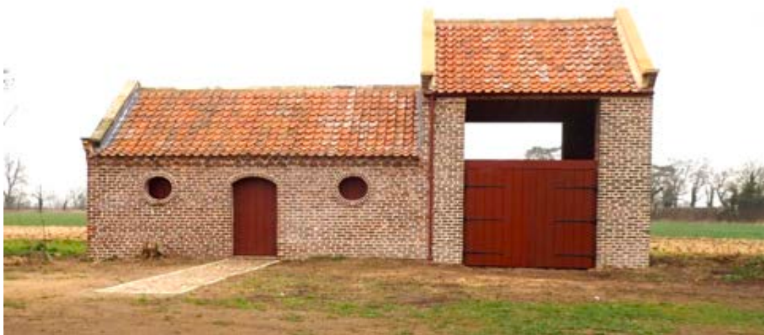
Nawton Towers, Pockley. 1 year after repointing:
