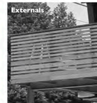
Timber balustrade to link between the house and parking area
