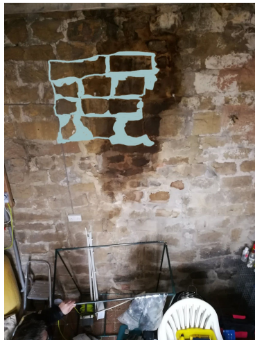
Fig 7 - Possible former aperture in former gable end, within byre
