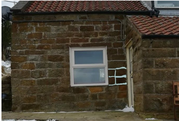
Fig 1 - Northern elevation showing possible filled aperture. Note the more regular and larger blocks on the top course of masonry
