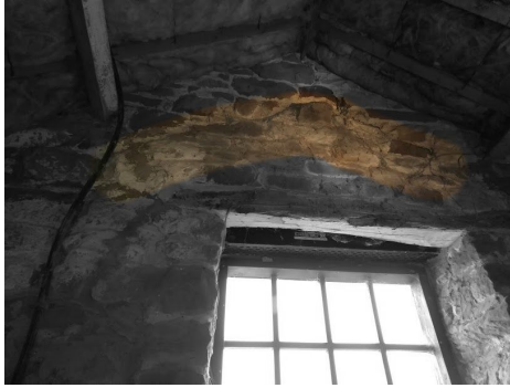
Fig 8 - Evidence of earlier roof slope in western gable
