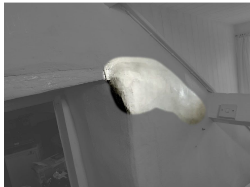
Fig 6 - Indication of earlier roof slope in dividing wall
