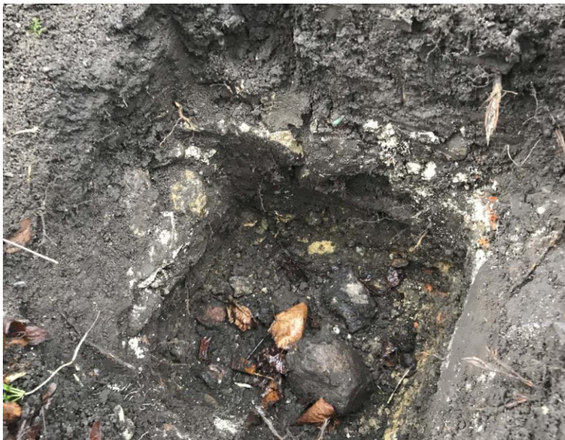
Photo 4 - Test excavation hole on access driveway
