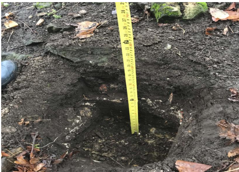
Photo 5 - Test excavation with tape for reference
