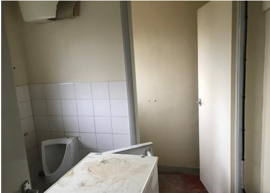
Figure 5: The interior – the former loos.
