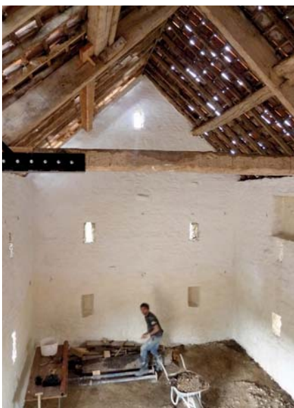
Hot lime washing in a threshing barn at Thornton Dale (Photo: Sam Baxter)
