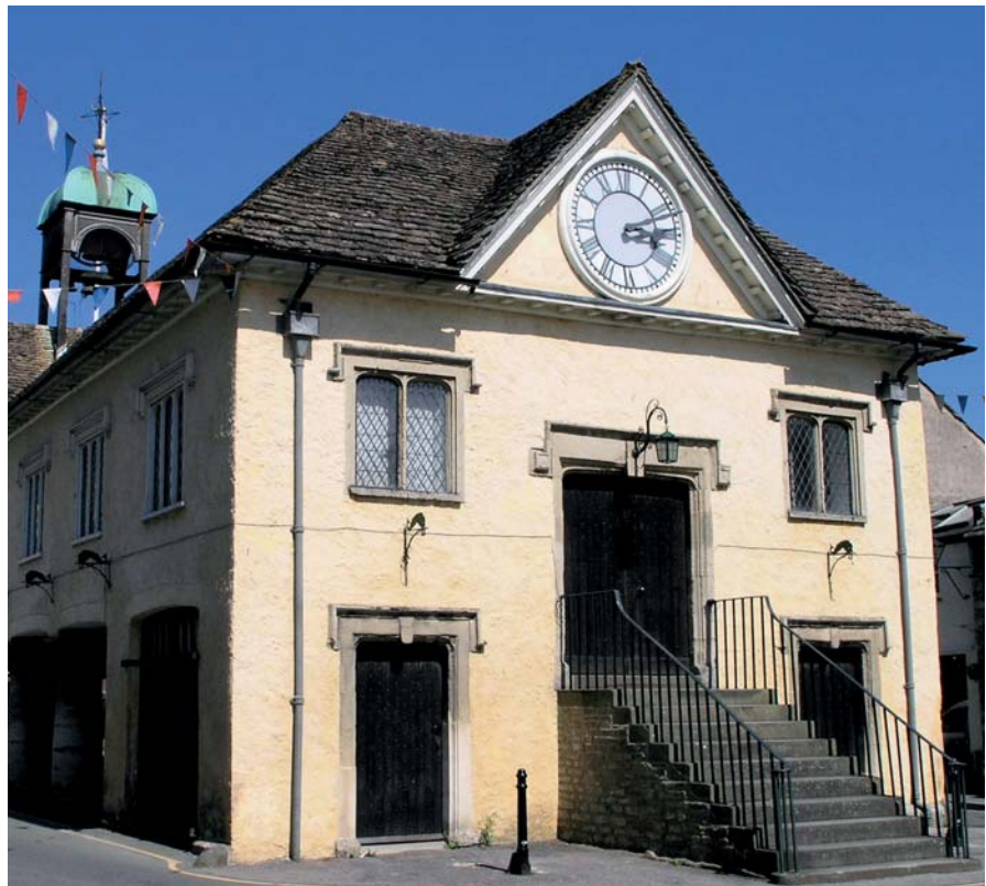
Traditional thick limewash on Tetbury Town Hall
