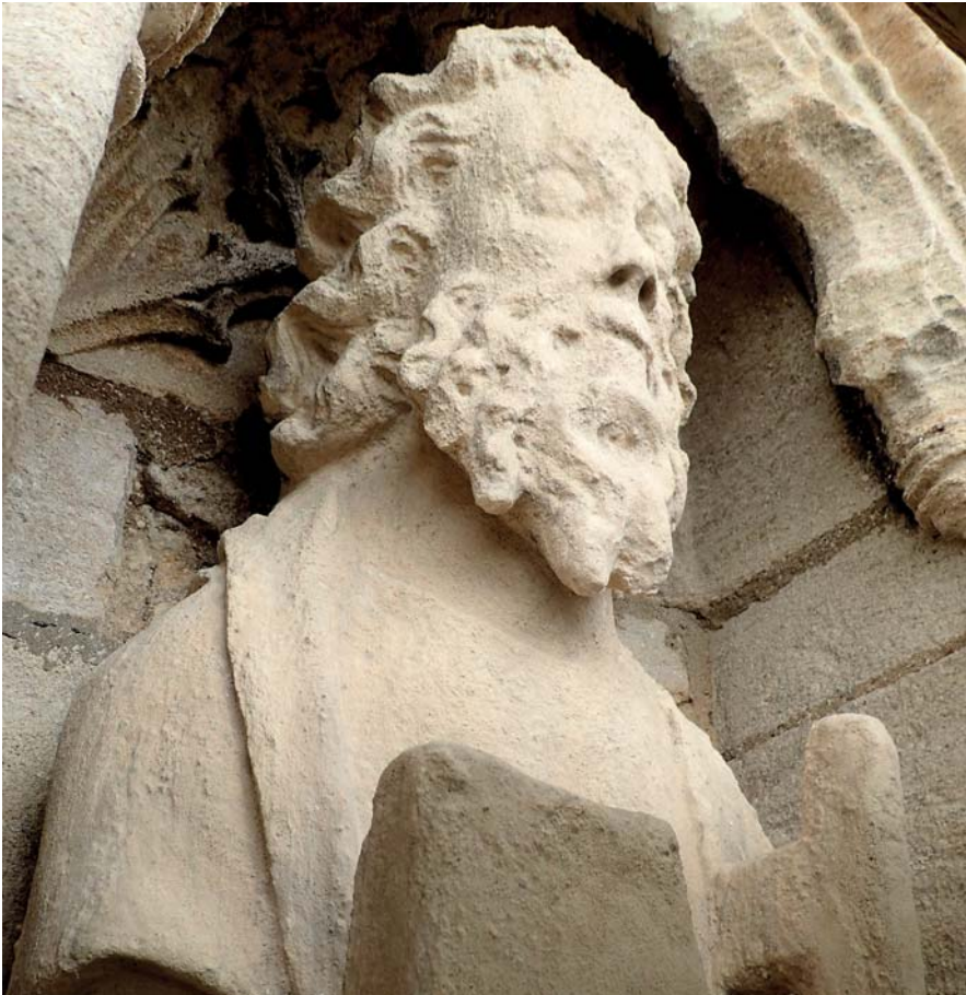
Recent conservation to the figures at Crowland Abbey church, Lincolnshire by Alex Carrington using hot-mixed mortars and shelter coats
