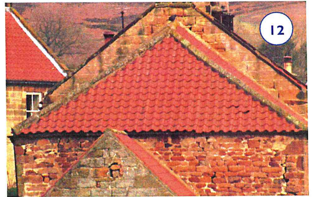
View of Cart house Wall External West Elevation
