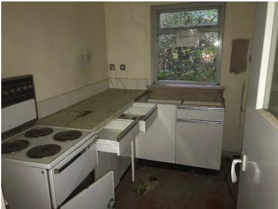
Figure 4: The interior - The existing kitchen.
