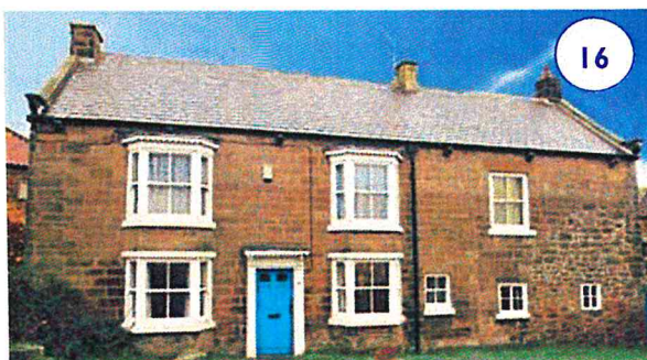
Osmotherley Listed Building - example of raising outbuildings in height
