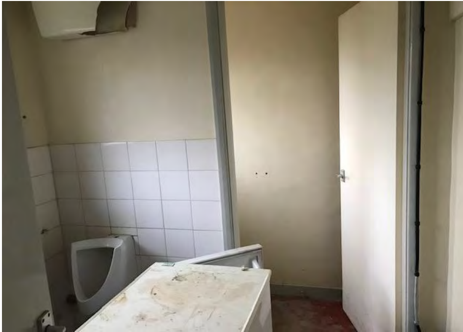
Figure 5: The interior – the former loos.
