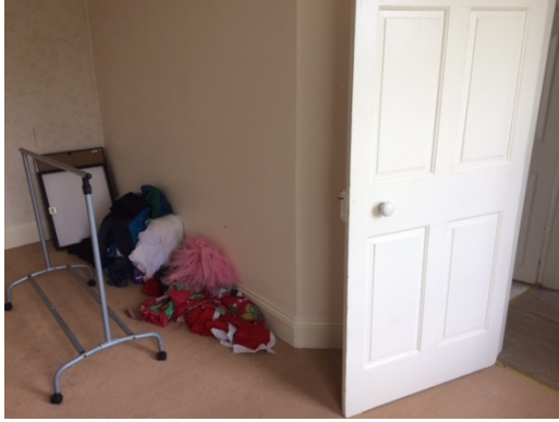
Image of existing modern stud partition with existing door (to be reused)
