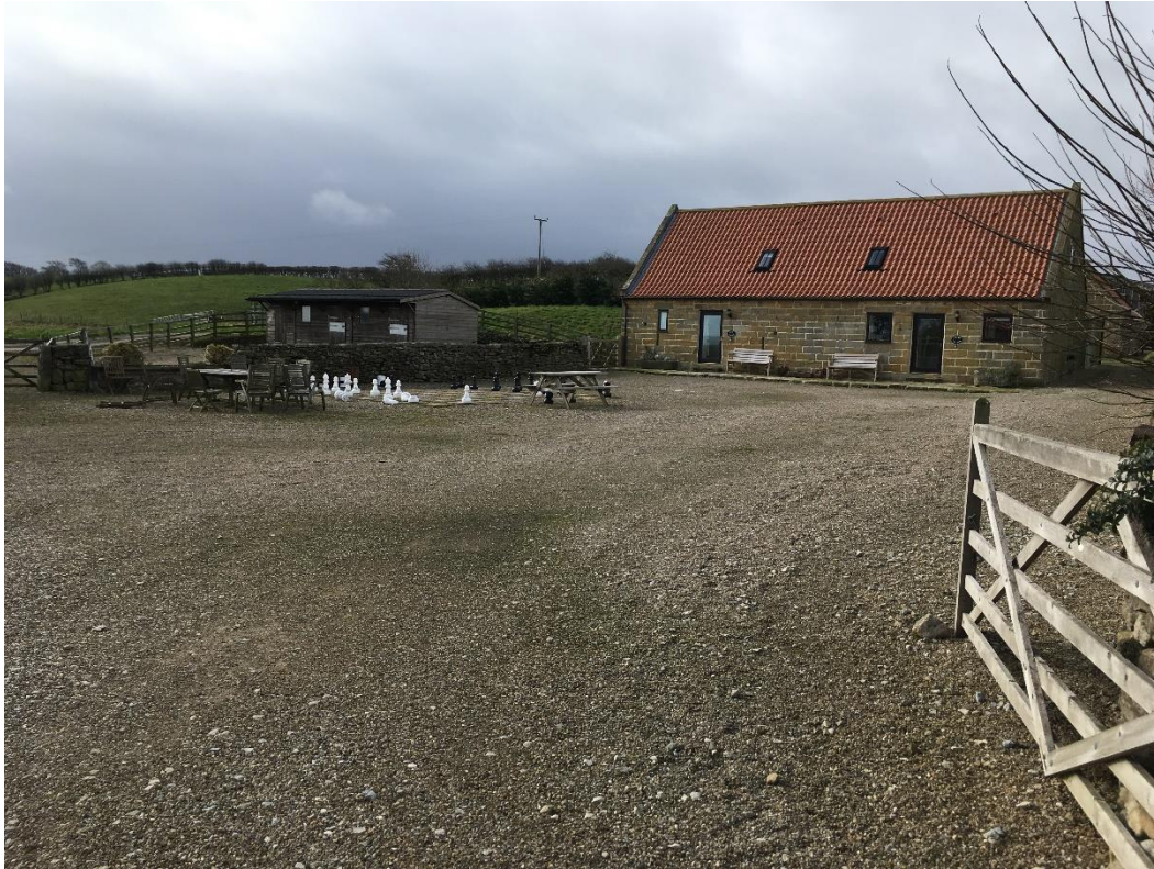
Fig 3. – Building 1 – future local occupancy dwelling
