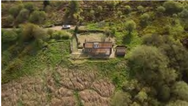
Fig 3. – overhead shot of the property and existing ‘concrete skirt’
