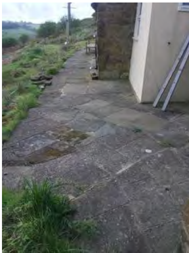
Fig 4. – shows existing the concrete apron
