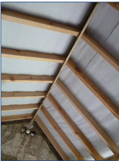
Photo 10: Internal roof and liner.
