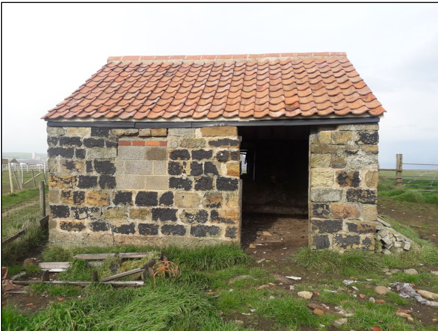
Photograph 3 – showing the front elevation (Elevation A)
