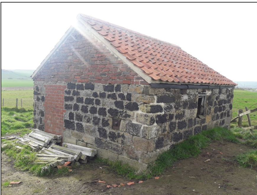
Photograph 1 – showing the side elevation (Elevation D) and rear elevation (Elevation C)
