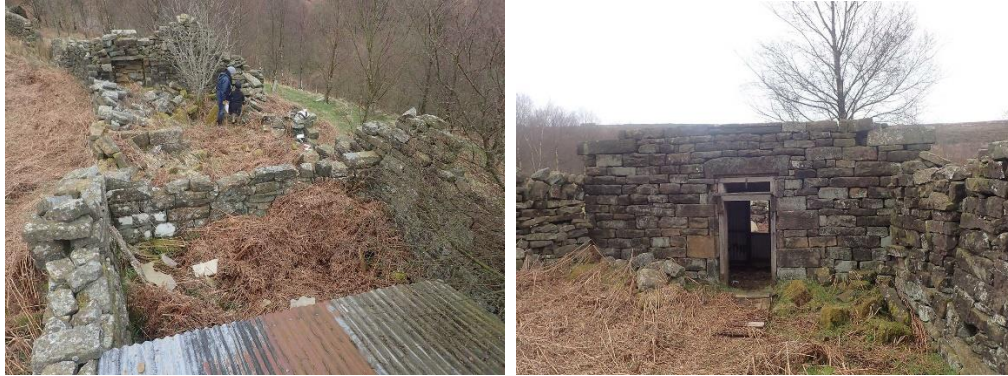
Figure 2.3 – Images of existing Red House site
