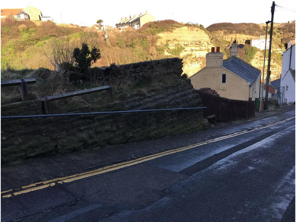
Photograph 1 East elevation and road (Staithe Bank)
