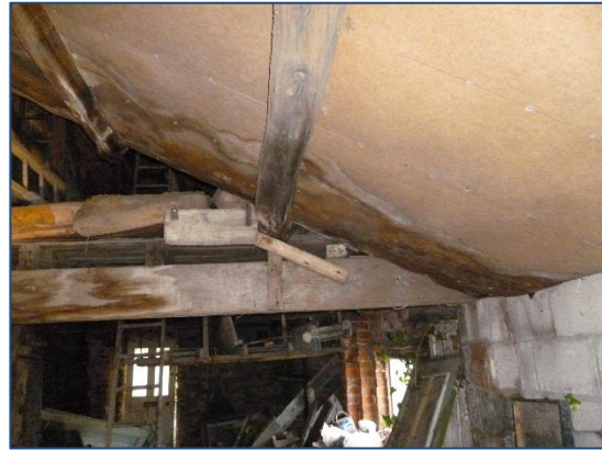
Photo 5: Section B mezzanine and lower floor, view from section A.
