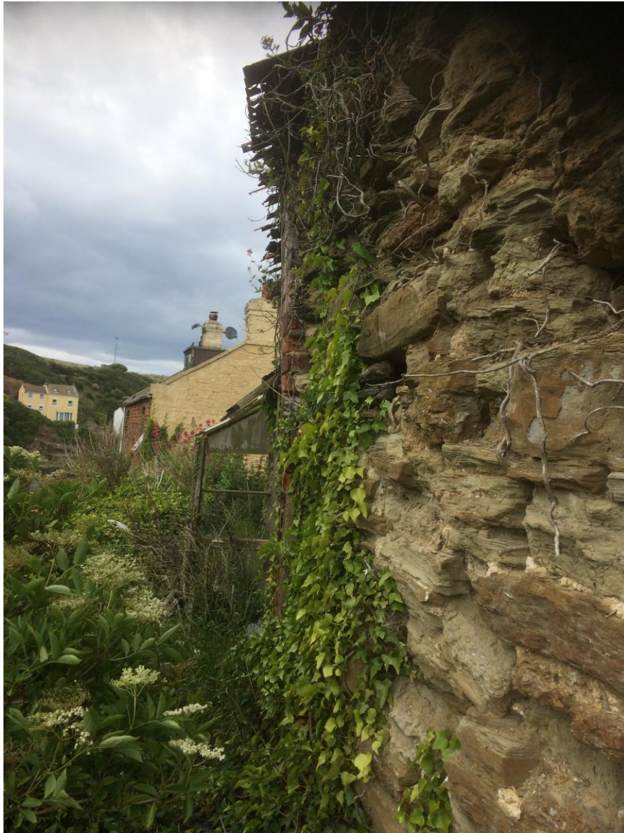
Photograph 4 The Olds Blacksmiths, Staithes Lane, Staithes
