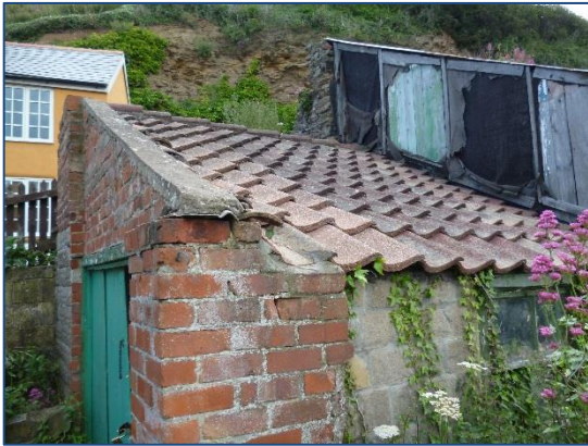
Photo 2: Section A northwest aspect.
