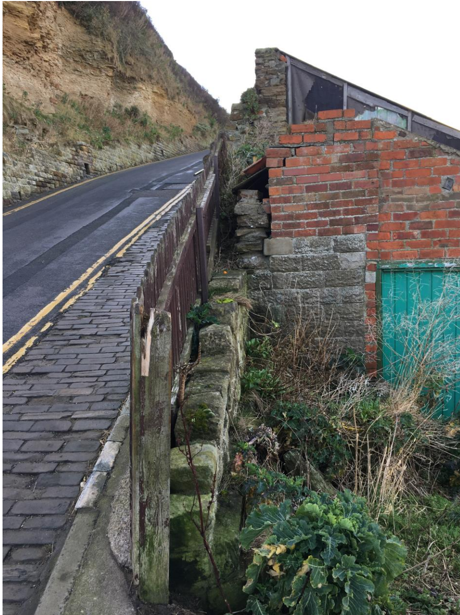
Photograph 5 The Olds Blacksmiths, Staithes Lane, Staithes
