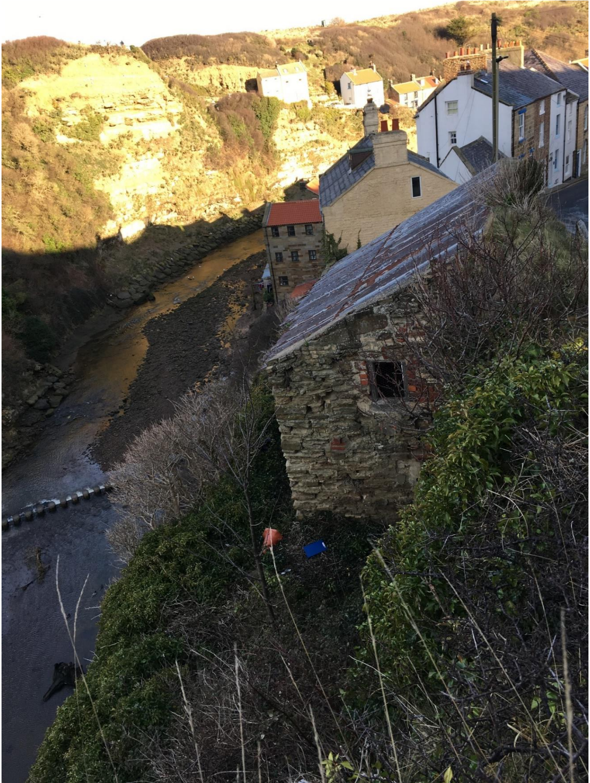
Photograph 2 South elevation looking north along Staithes Beck
