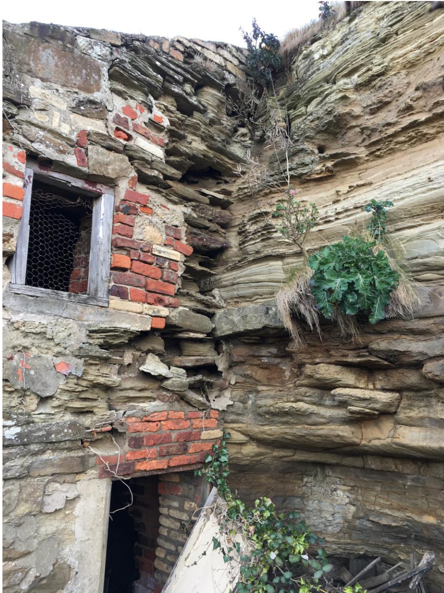
Photograph 7 The Olds Blacksmiths, Staithes Lane, Staithes
