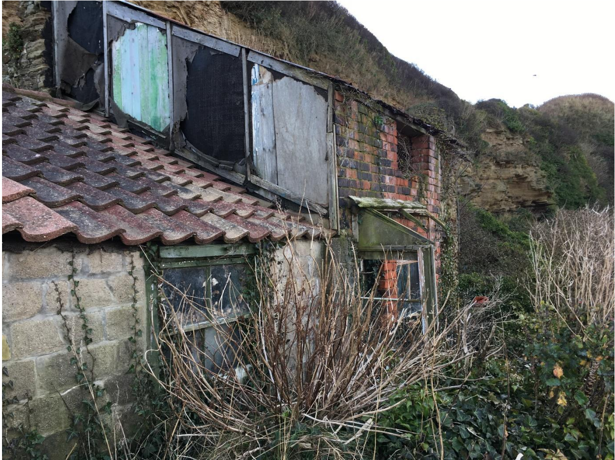
Photograph 3 West elevation, note remnants of timber porch
