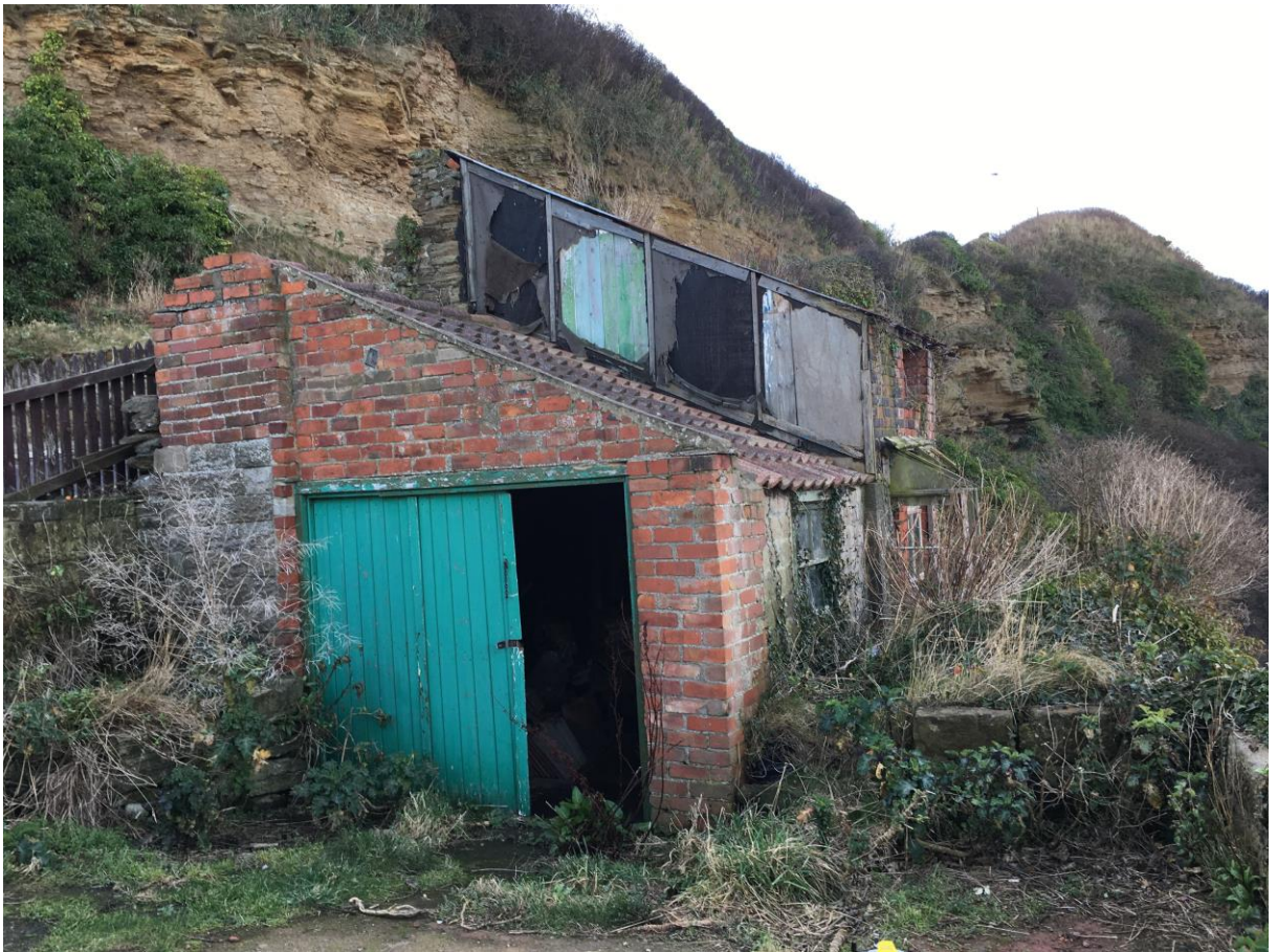
Photograph 1 The Olds Blacksmiths, Staithes Lane, Staithes
