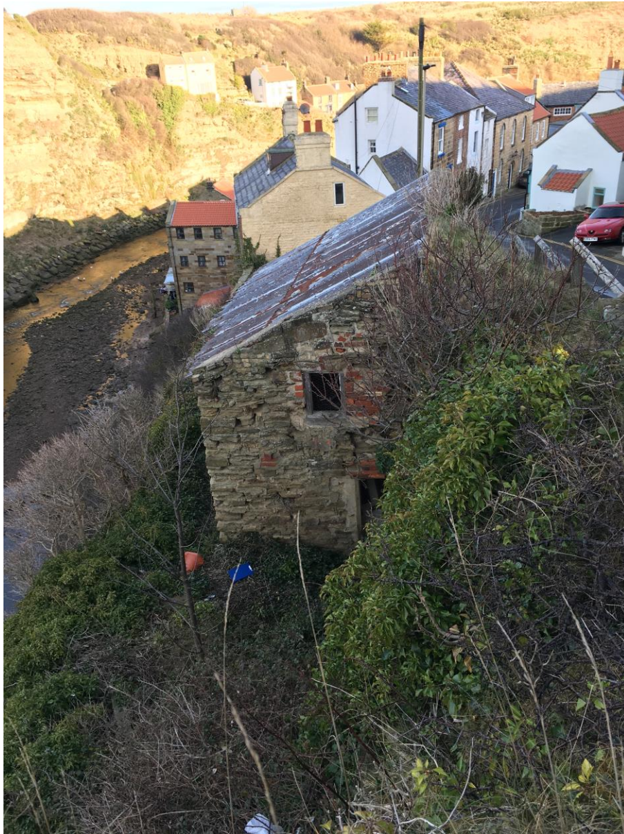
Photograph 6 The Olds Blacksmiths, Staithes Lane, Staithes
