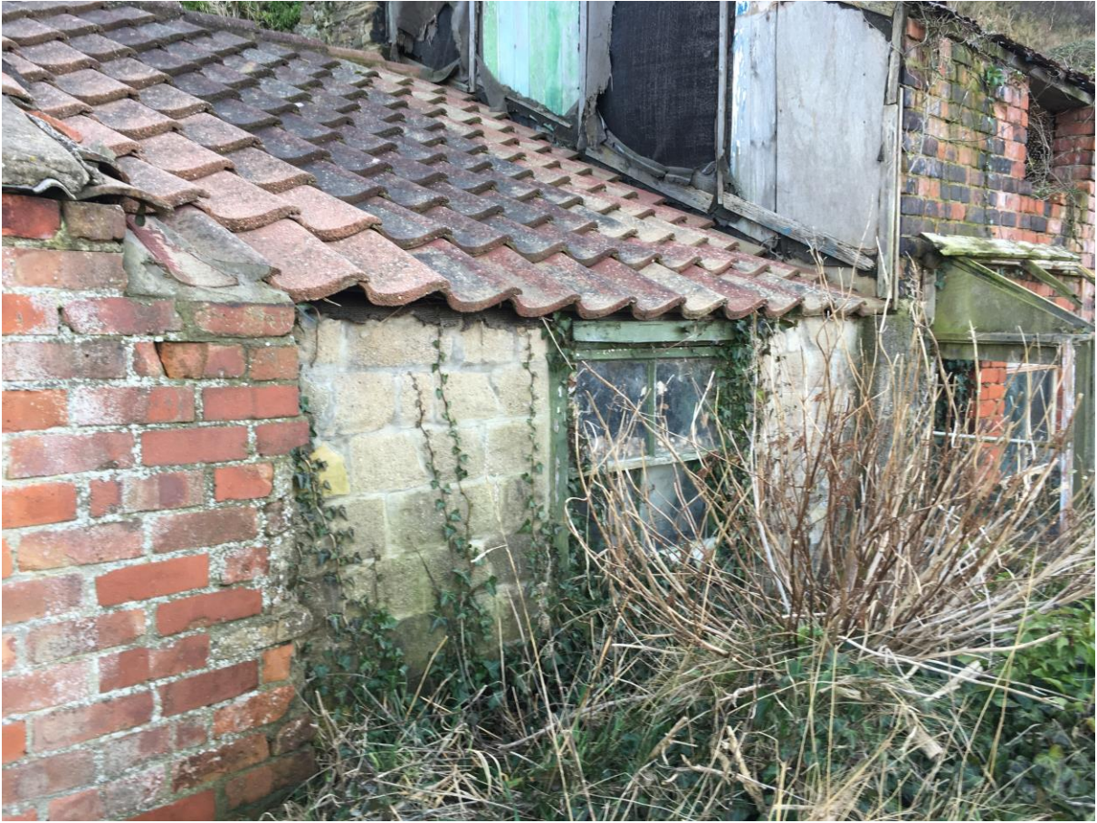
Photograph 2 The Olds Blacksmiths, Staithes Lane, Staithes
