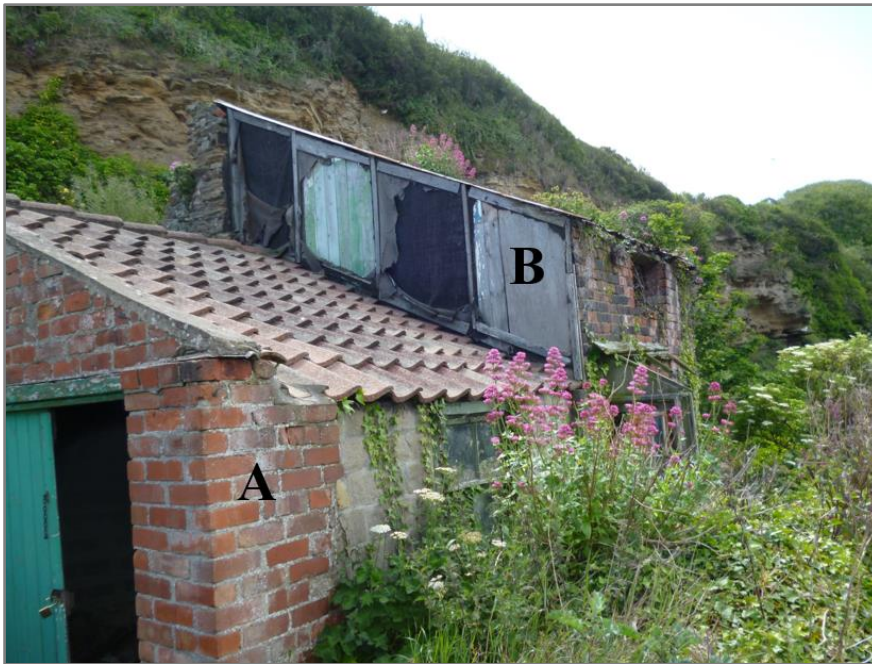
Photo 1. The Old Blacksmiths, southwest aspect.
