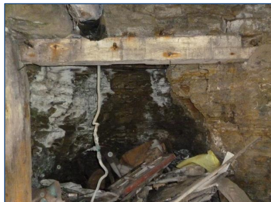
Photo 7: Section B cliff side wall.
