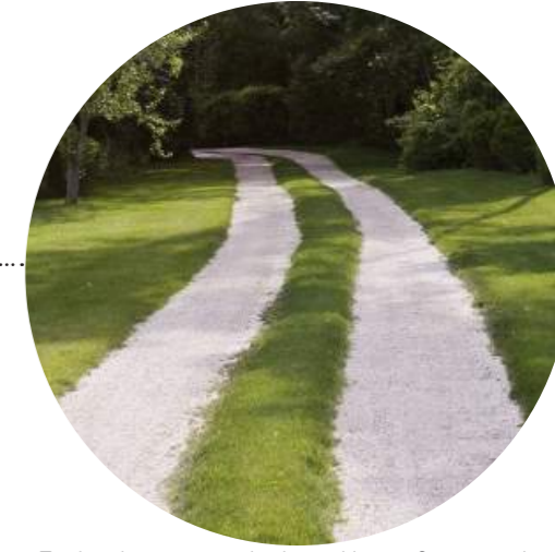
Existing track leading from the main quarry road to be stone wearing strips with central grass strip
