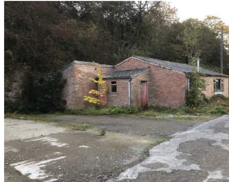
Existing quarry canteen
