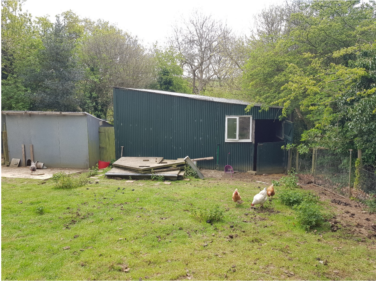
North elevation of existing outbuilding.
