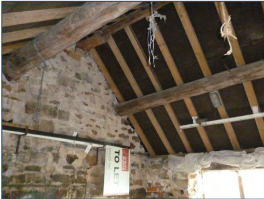
Photo 4: Wooden beams and lined room in room A.
