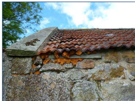
Photo 7: Expanding foam filling gaps in eaves on roof of room B.
