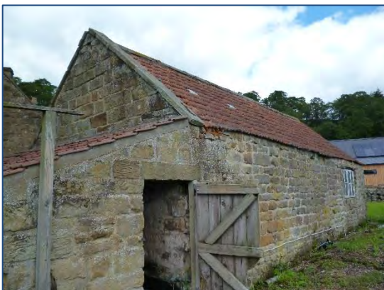
Photo 6: SE side of building with door to room C.
