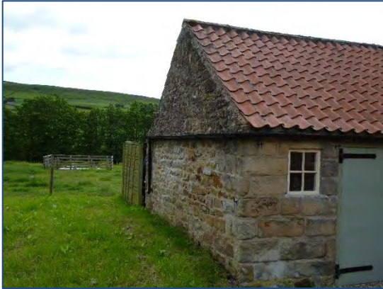
Photo 2: NW aspect with well-sealed stone-work and door to room A.
