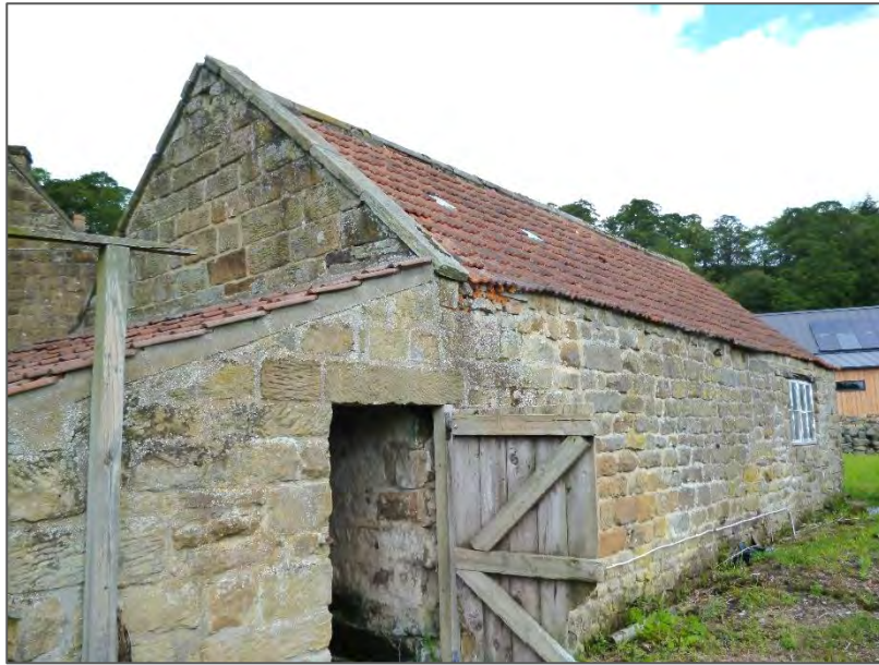
Photo 1: South-east aspect of the outbuilding at Church Houses Cottage.
