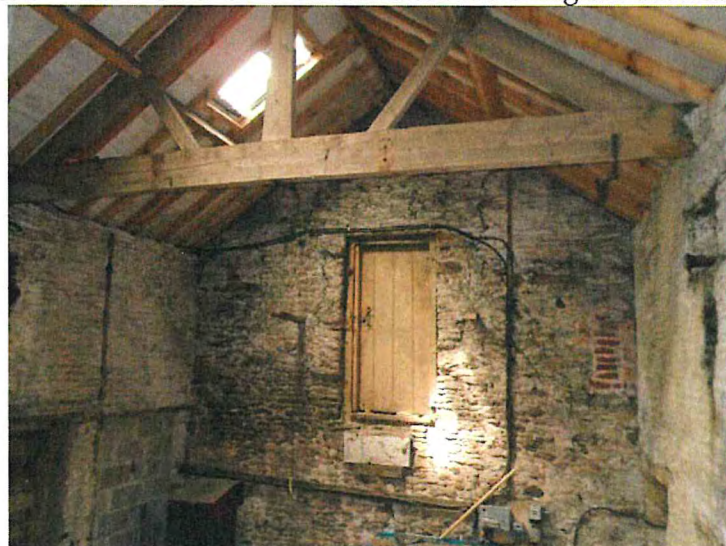
Plate 3 – internal section to be converted into living accommodation.
