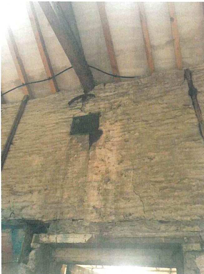
Photograph 17 – cracking over timber lintel below truss seat
