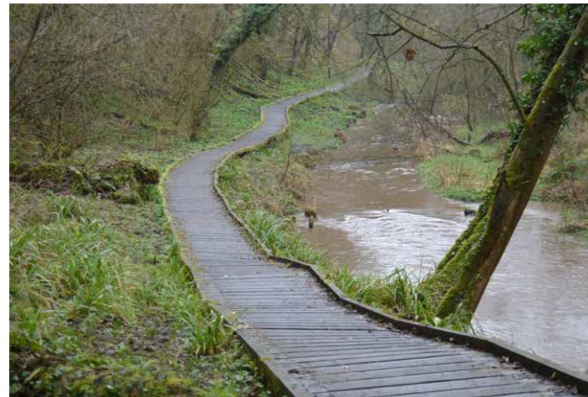
Context photos showing the existing footbridge
