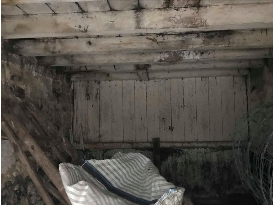
Image 5. Internal of central store room
