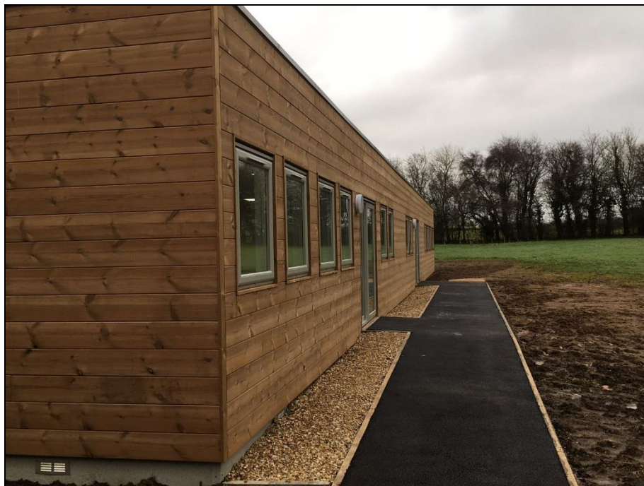
Figure 3 – indicative image showing Thermowood horizontal cladding
