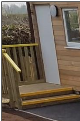
Figure 5 – indicative steps leading from fire exit
