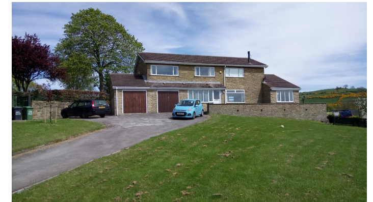
View Of Existing House
