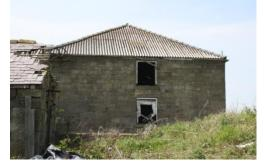
2.13 To the rear of the granary lie three large shelter sheds formed of the original two wings to the farm and a later inserted overall roof which created a large open space for stock but has now collapsed throughout most of its length. This group of structures is noted as number 7 on the identification plan. The eastern wing has a brickwork inner wall and good quality cut and dressed
