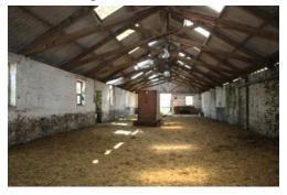
stonework walls to the east and south elevations. The roof is supported on timber scissor trusses and has a corrugated sheet roof with panels of clear corrugated sheeting to light the interior. Internally any divisions have been removed to create a large shelter shed for livestock. The internal, western wall to the courtyard has no openings however the eastern external
