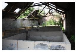
2.16 To the east of the principle outbuilding lies building 3, the piggery. This is another stone building of matching construction to the better quality buildings on the site and for the most part this retains its slate roof which has raised
