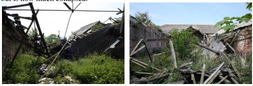
2.15 The western wing mirrors its eastern counterpart in scale and form however with certain important differences. The roof is a lightweight steel and timber construction matching the remains of the central section, and this too has
