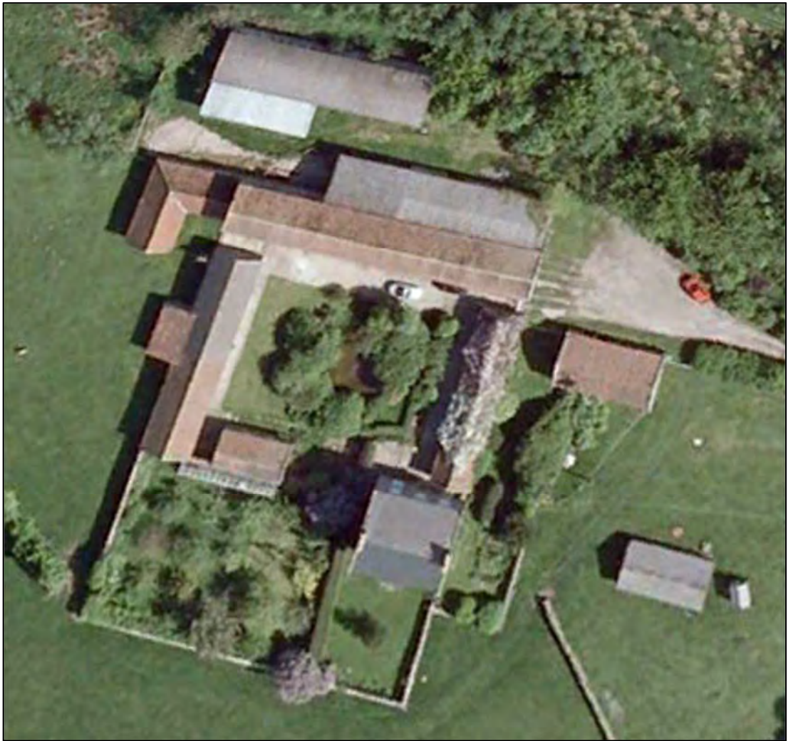
Figure 9: historic Google Earth imagery (2009) of Thirley Cotes farm prior to its development as holiday accommodation. The demolished 'greenhouse' building is visible extending to the rear of the south range. Also visible are a series of modern agricultural building with corrugated roofs, all of which have since been demolished.
