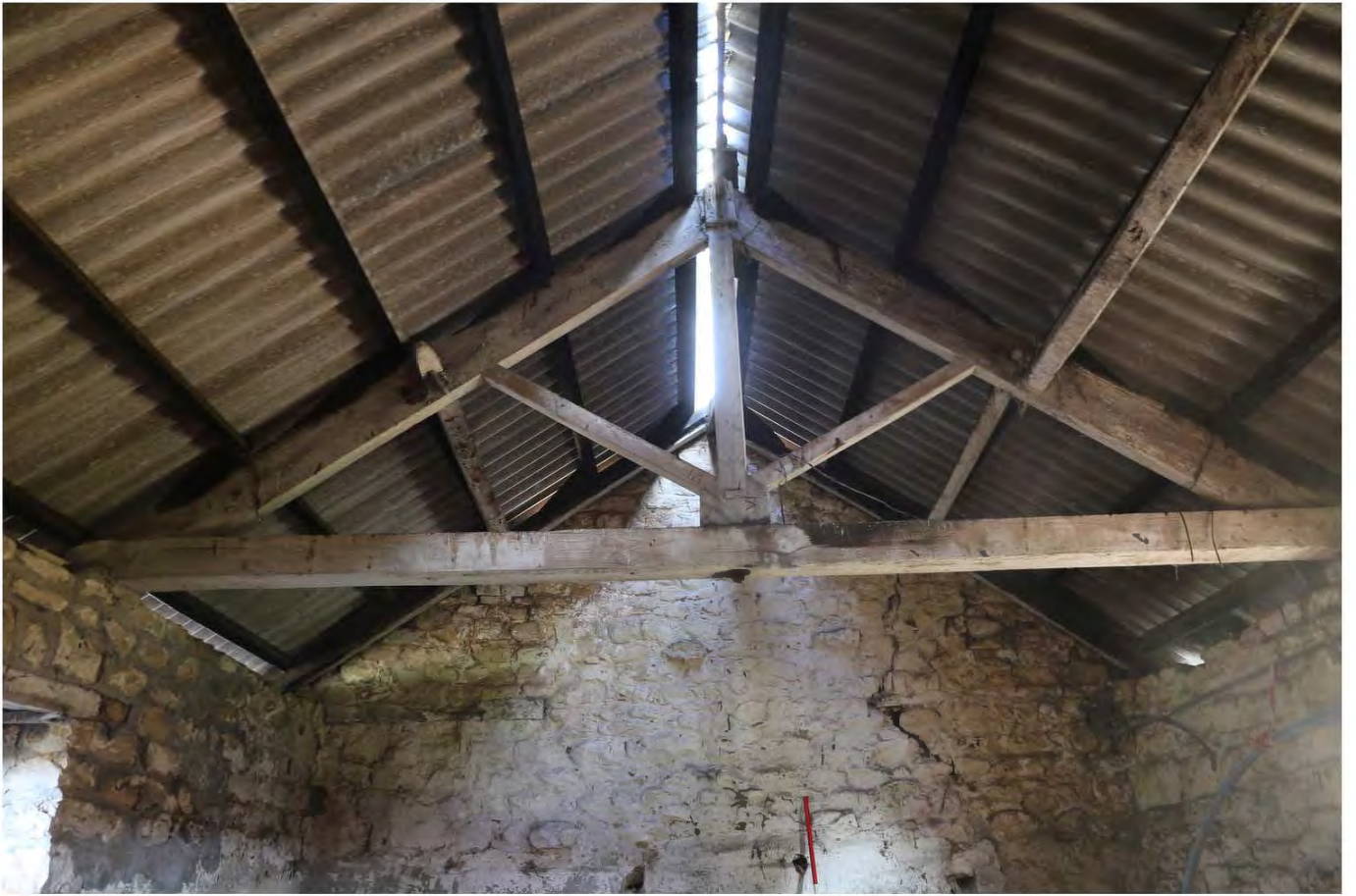
009_100_108_truss lk N
