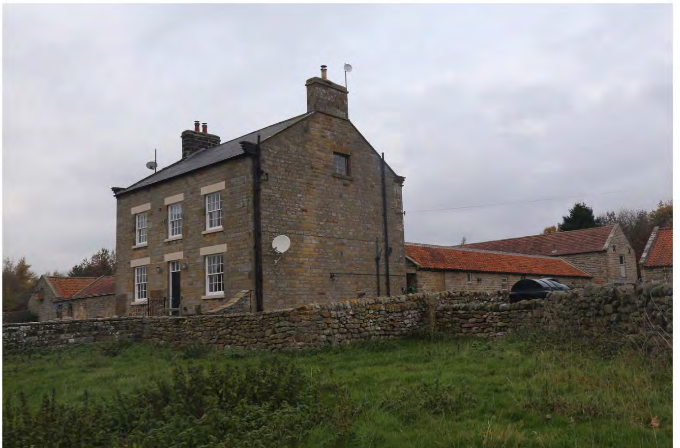
113_Gen_view of_house oblique lk NW - East gable
