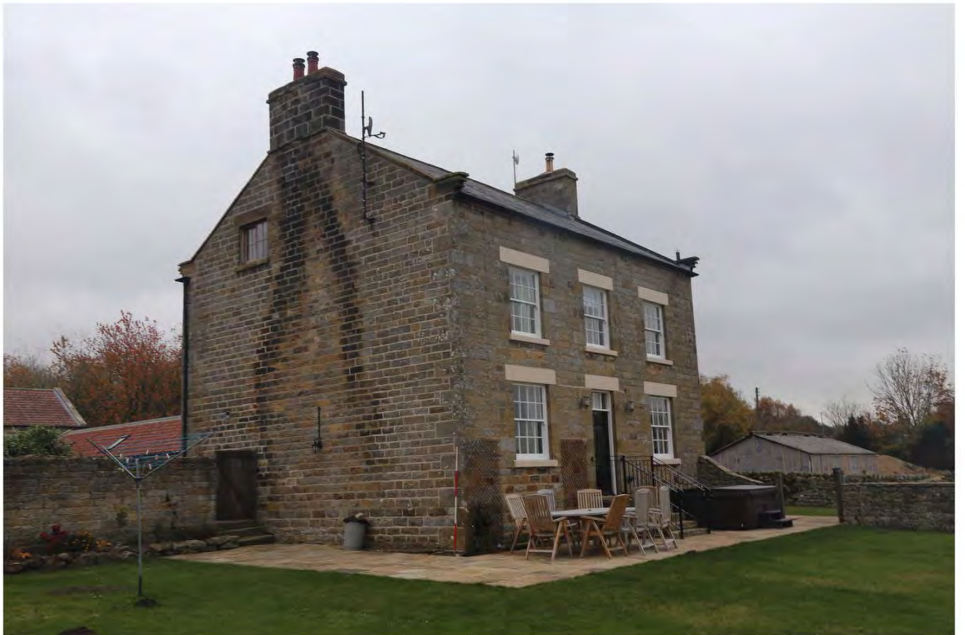
115_Gen_view of_house oblique lk NE
