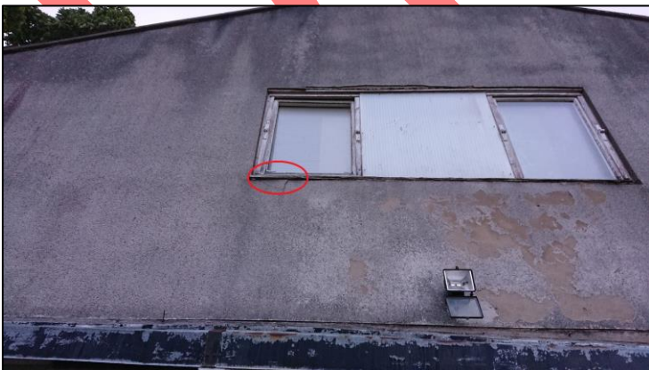
Figure 65. Common pipistrelle roost entrance
