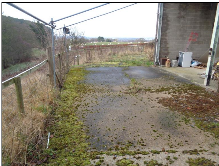
Figure 17. Hardstanding next to the south eastern elevation
