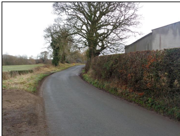
Figure 11. Dikes Lane looking north; the building and sycamore (TN2) can be seen
