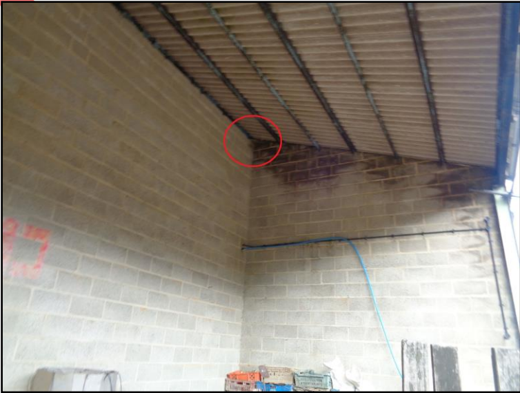
Figure 33. Open barn on south eastern elevation. Remnant bird's nest and potential bat roost entrance marked
