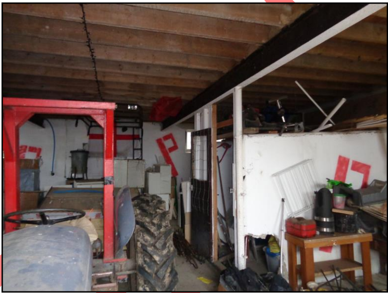
Figure 38. Main room on the ground floor
