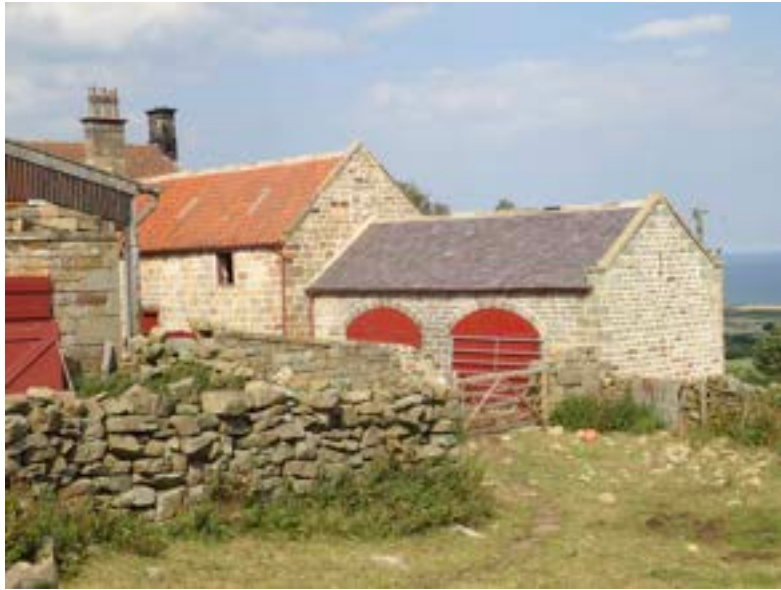
Scampston Hall, 18thC horse shelter and cart-shed, 1 months after repointing:
