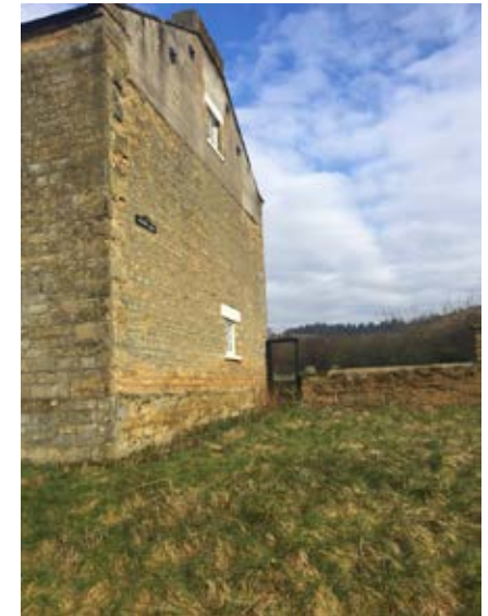
East elevation of existing house
