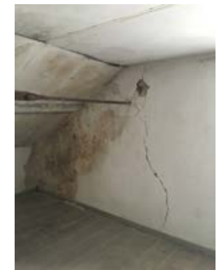
Attic room (note tie rod)
