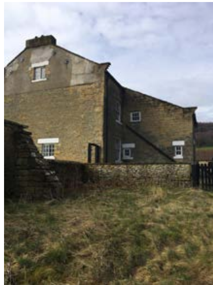
East elevation of existing house
