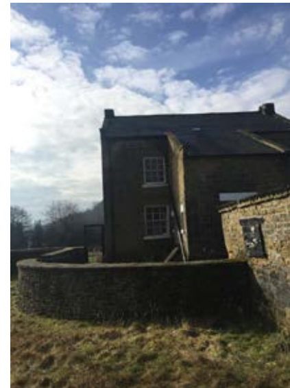
Rear (north) elevation of existing house
