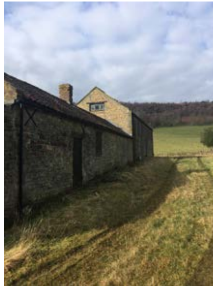
North elevation of northern range
