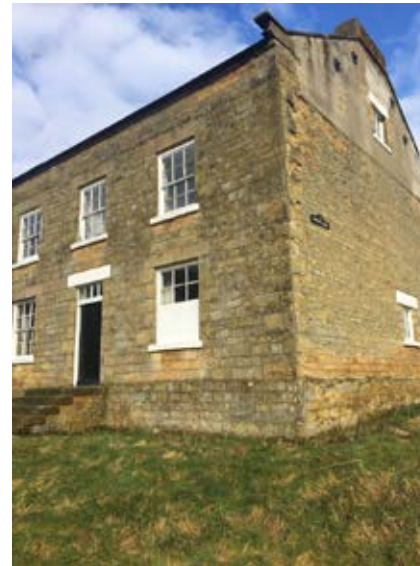
Front (south) elevation of existing house
