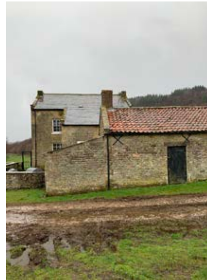
North elevation of northern range (rear of existing house behind)
