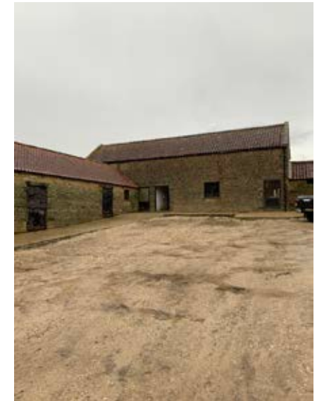
South elevation of two-storey barn and east elevation of western range
