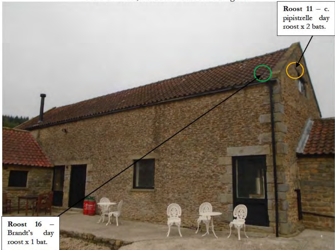
Plate 5 – barn, south elevation and east gable.
