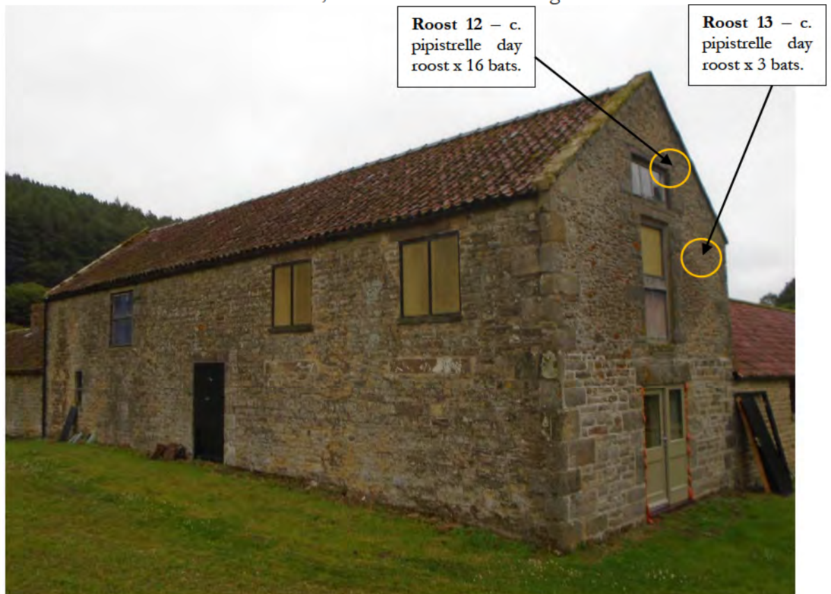
Plate 6 – barn, north elevation and west gable.
