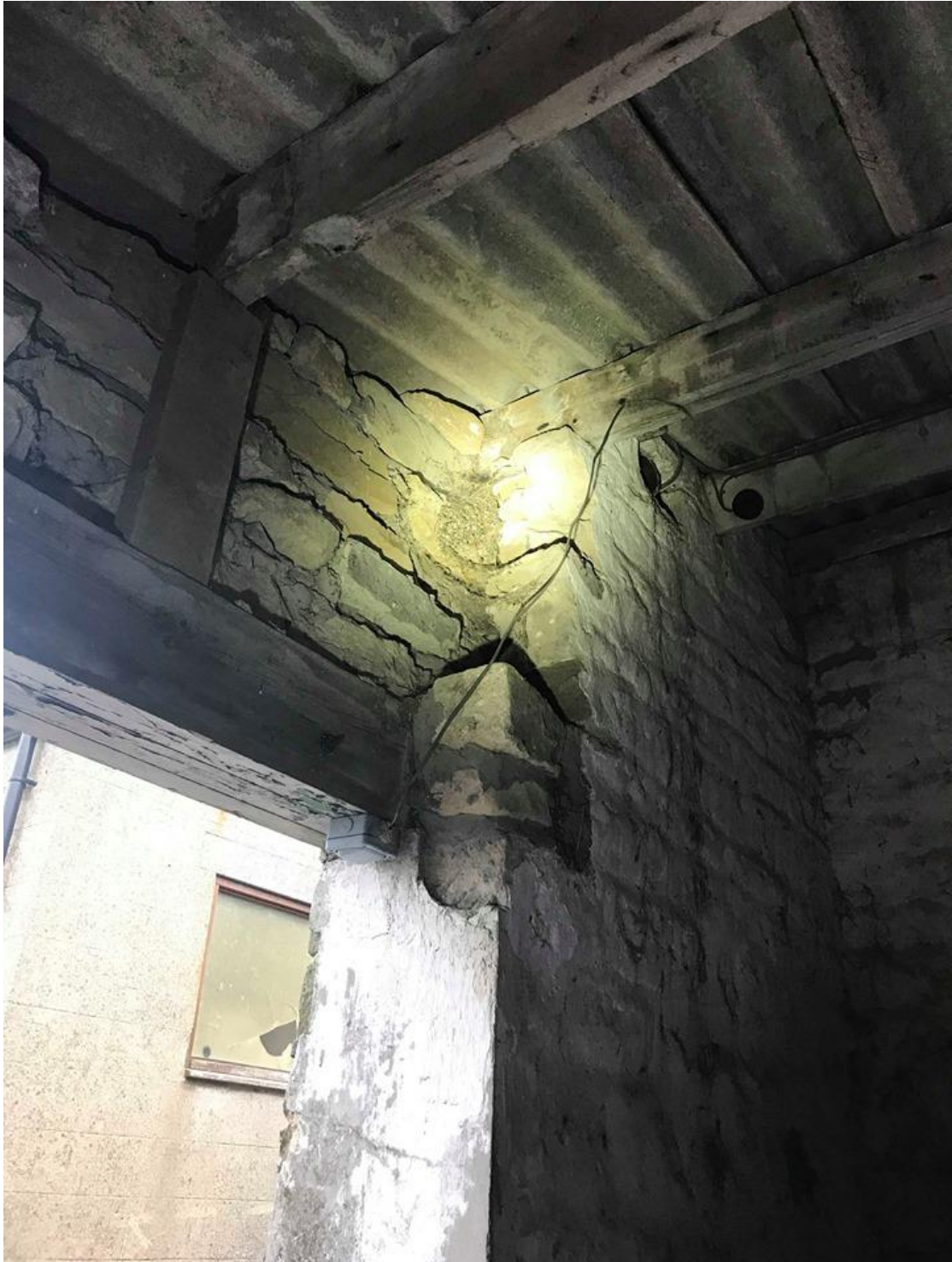
Image 6. Internal of open garage showing recently used bird nest
