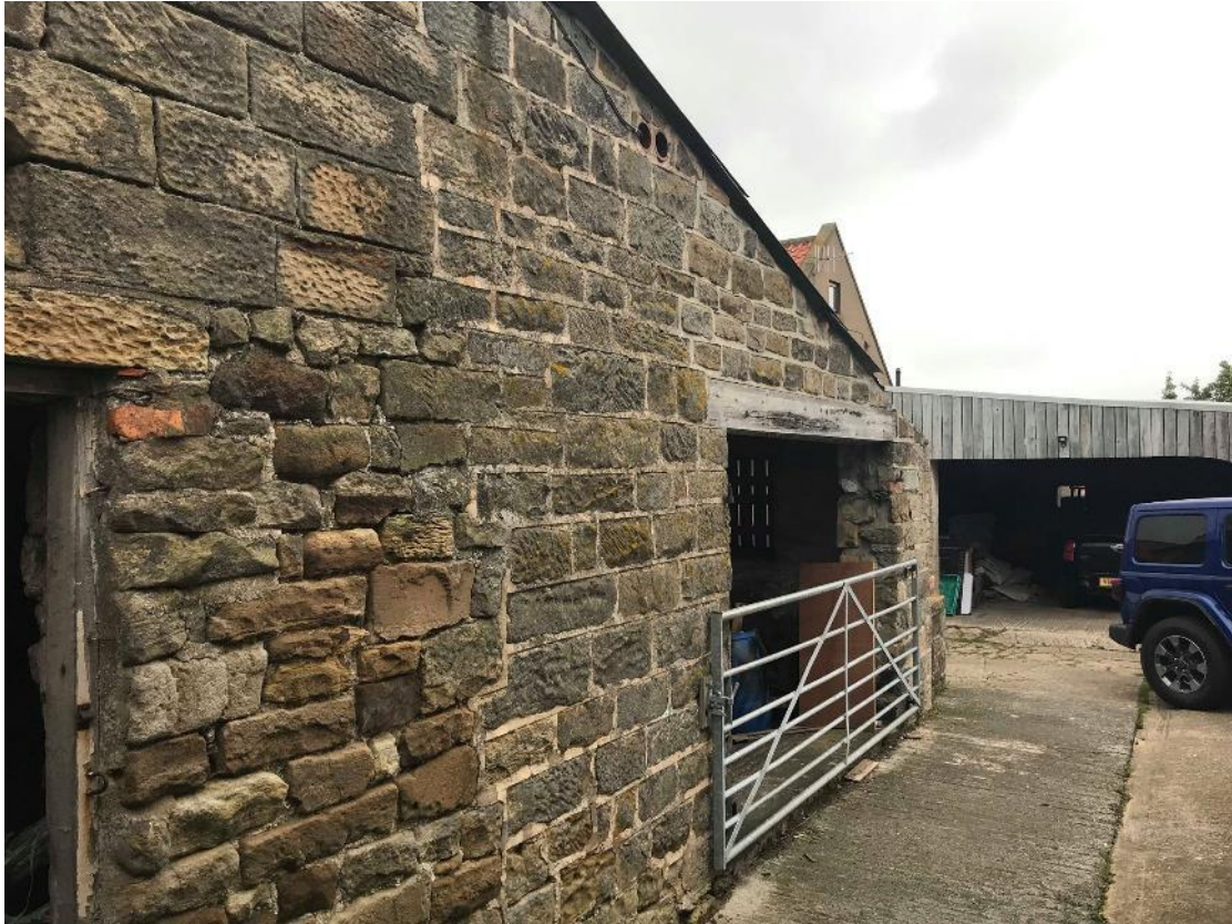
Image 4. East elevation of target building.
