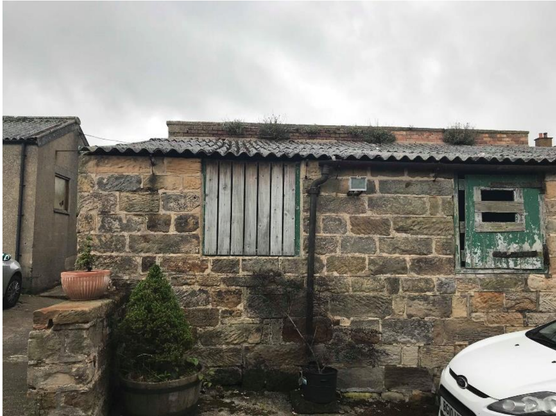
Image 1. North elevation of building
