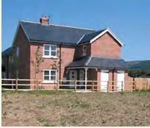
Affordable Housing, Battersby Junction
