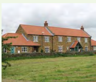
Affordable Housing, Egton
