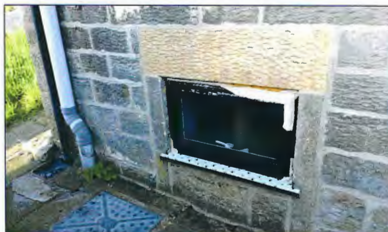
No1 Fairhead Cottage kitchen window
