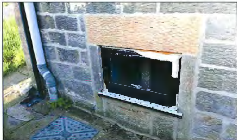
No1 Fairhead Cottage kitchen window
