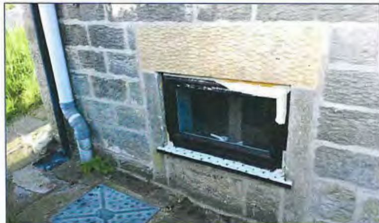
No1 Fairhead Cottage kitchen window
