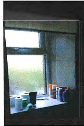
(Bathroom – First floor)
