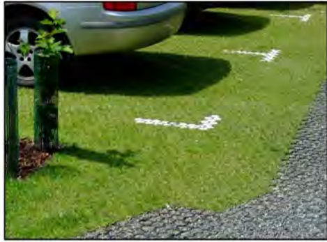
example of a Turf Reinforcement System - Geosynthetics Golpla
