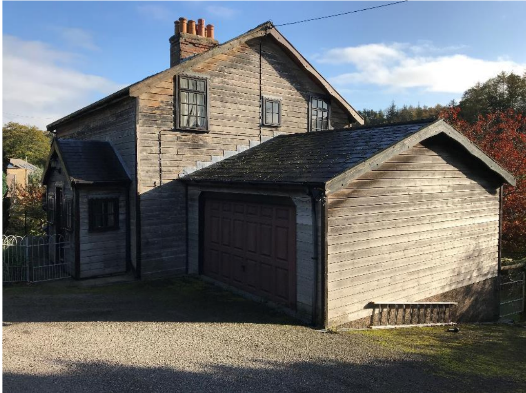
Image 1. Existing property, looking north-east.
