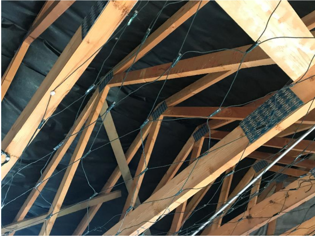
Image 4. Roof space of garage.
