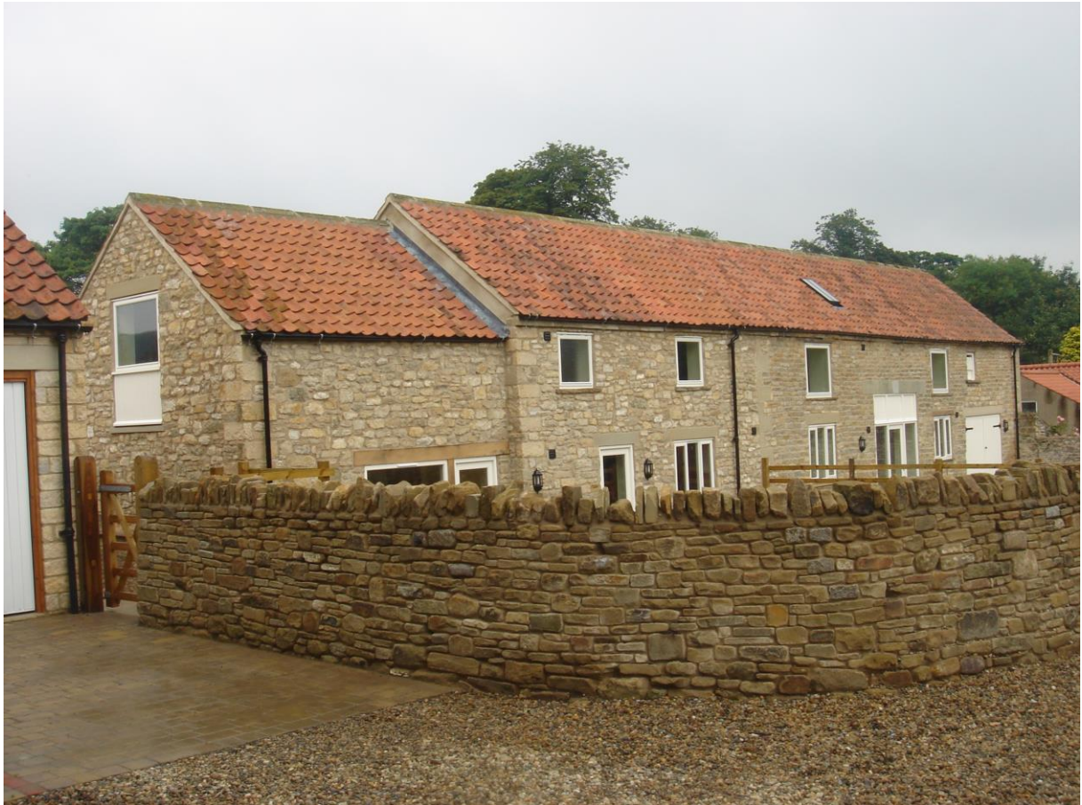
Originally two barns, this building has been converted and a small extension added to the left-hand side to form 2 cottages now known as 2 and 3 Brookfield Gardens.
