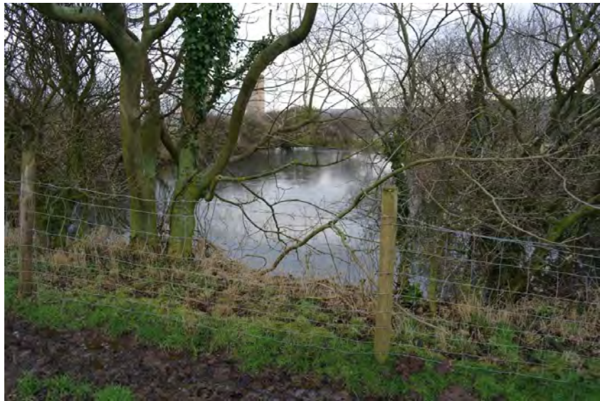
Boulby Ironstone Mine reservoir, to be retained as existing with stockproof fence surround and warning signs or remodelled with shallow edges as wetland habitat if long term public safety is a concern.
