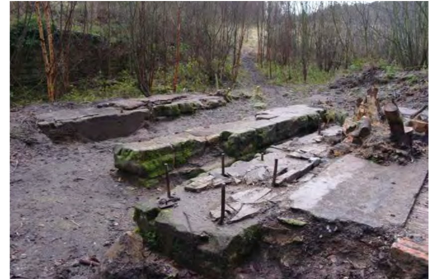
Grinkle Mine, remnant foundations.
