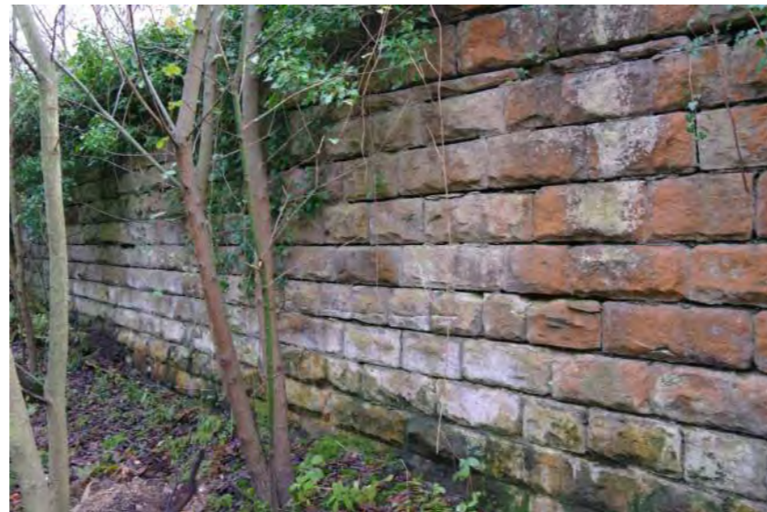
Grinkle Mine - remains of substantial masonry retaining wall.
