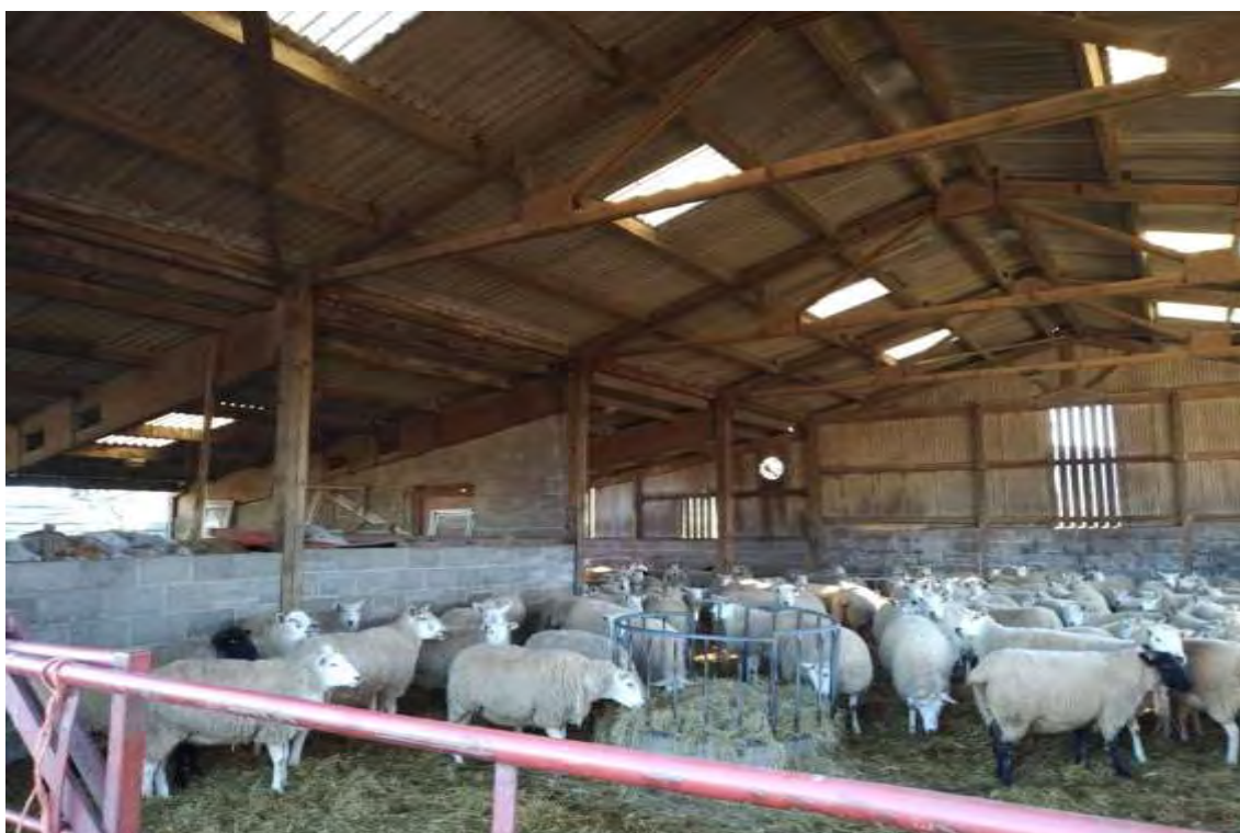
Photograph 22 Western part of Building 14, barn still intact and houses sheep.
