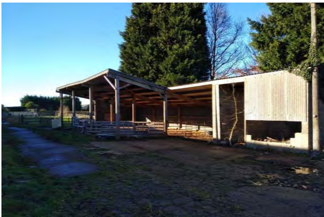
Photograph 1 Building 1 southern aspect.
