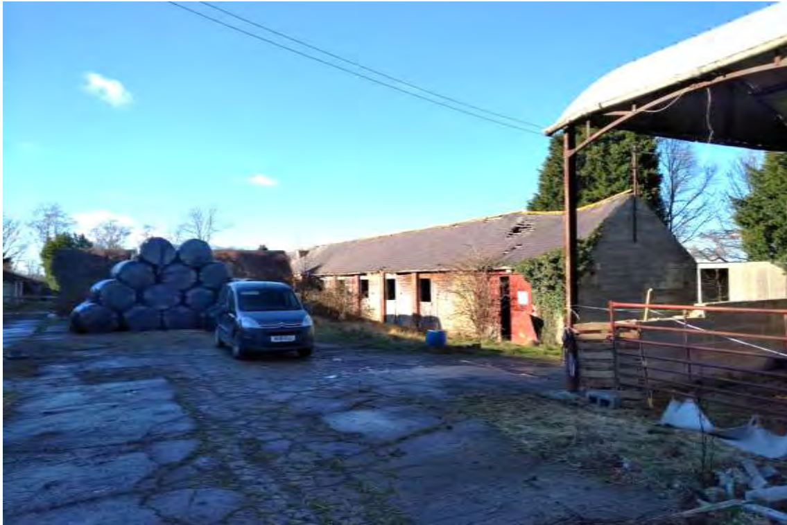
Photograph 3 Building 3 southern and eastern aspect.
