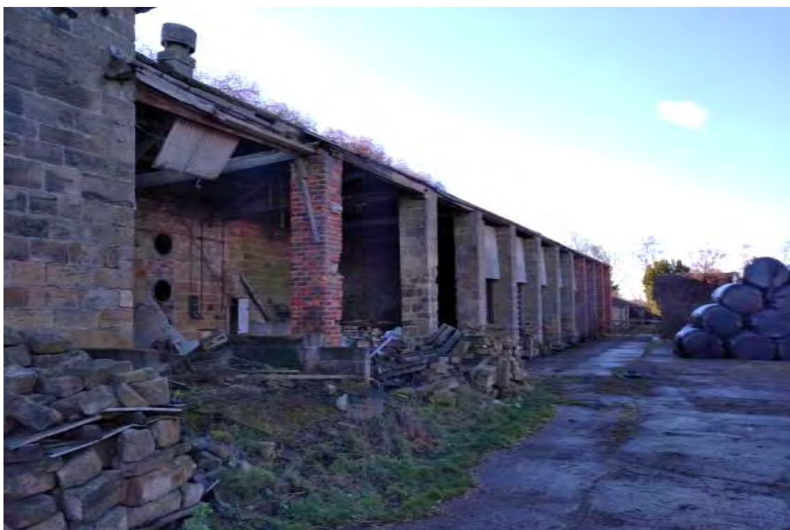
Photograph 6 Building 5, northern aspect.
