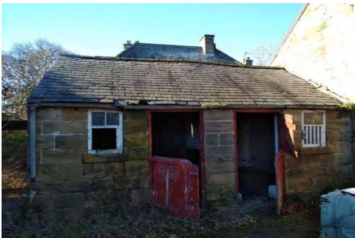
Photograph 18 Building 11 - still has opportunities for void and crevice dwelling bats.
