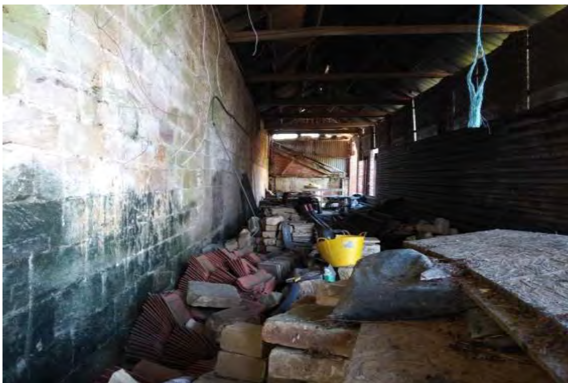
Photograph 7 Building 5 internal structure. Illustrating storage of reclaimed building materials.
