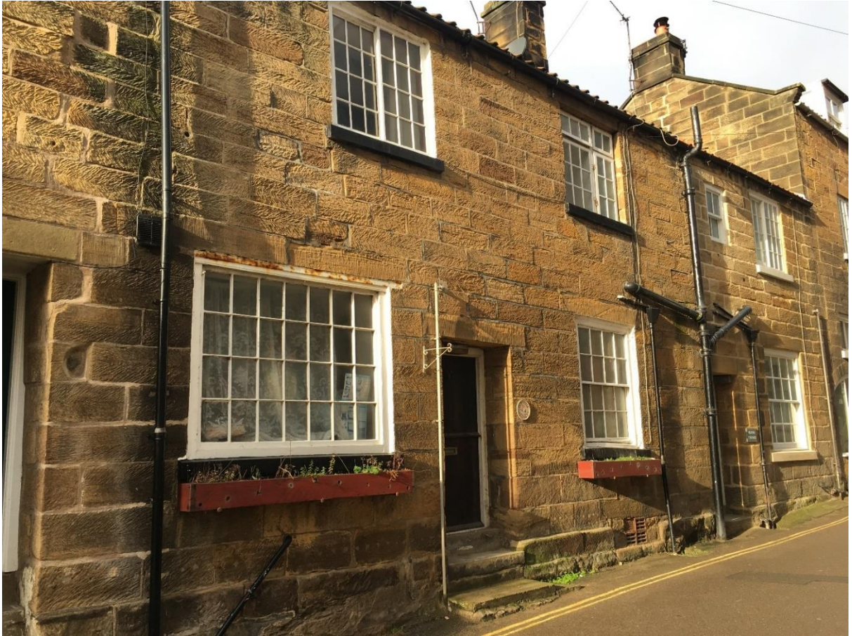
Photograph 7 Front elevation with Beadle Cottage beyond
