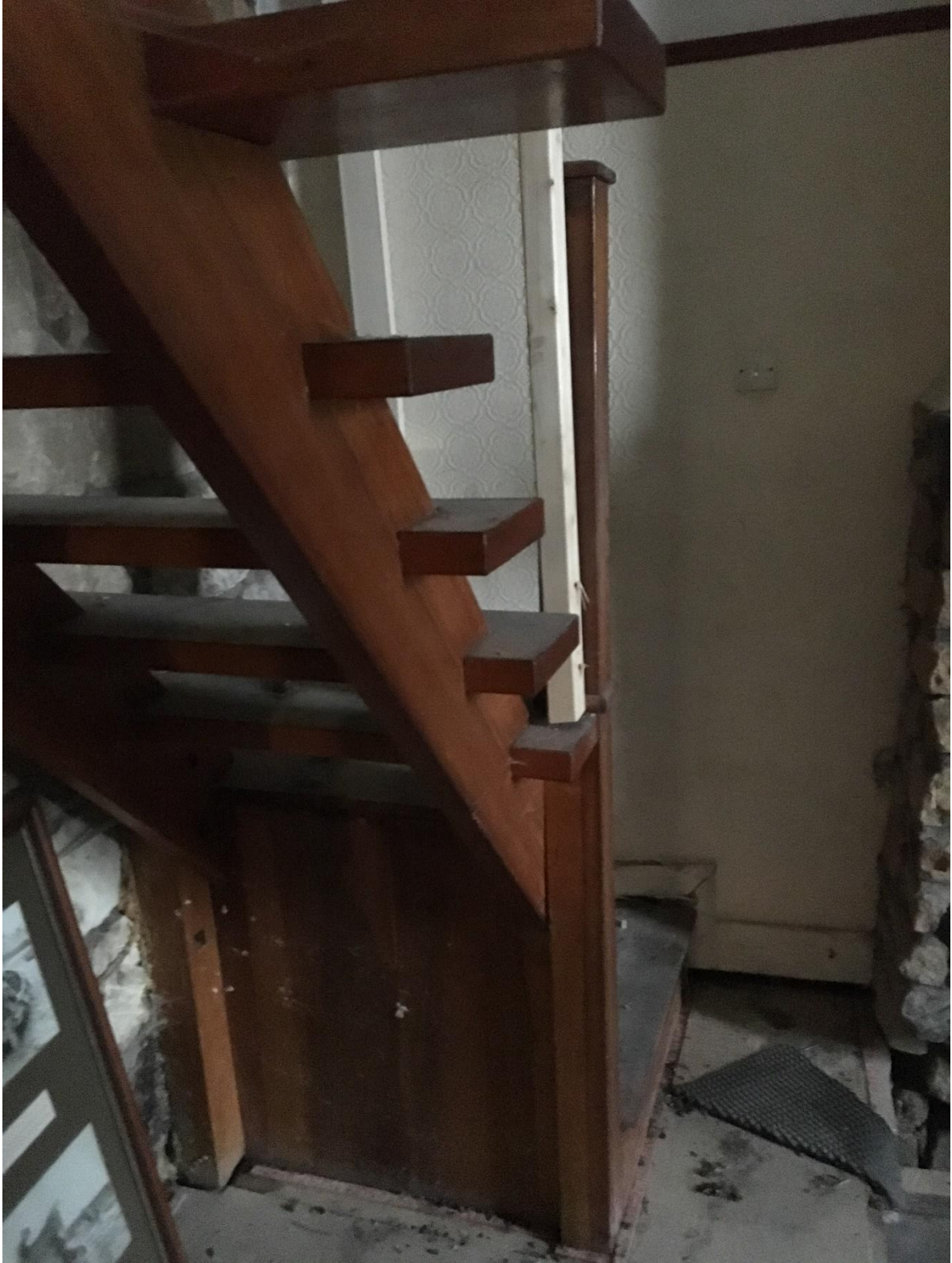
Photograph 2 Open plan stair to lounge
