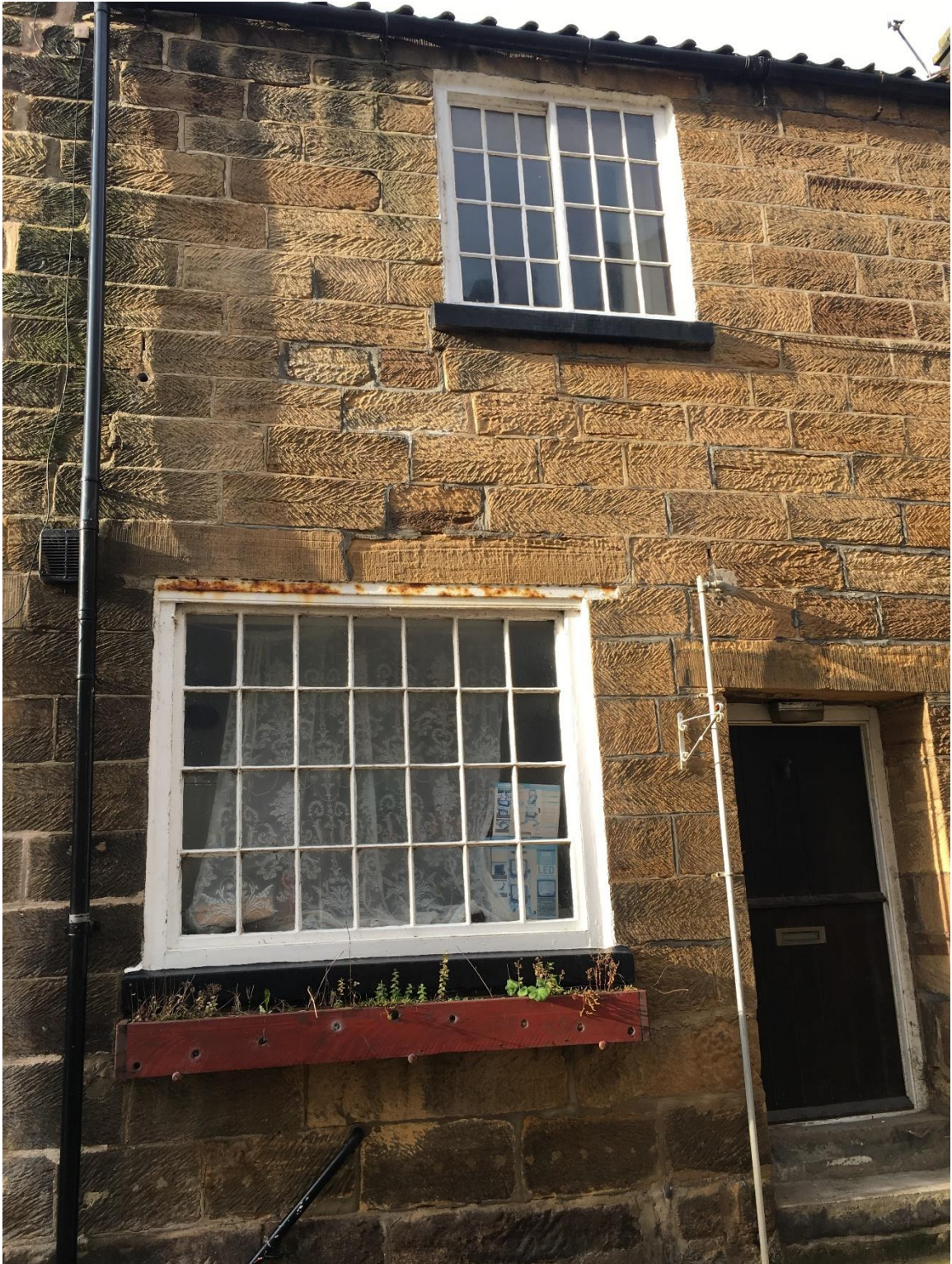
Photograph 5 Part Front Elevation, W1 and W3
