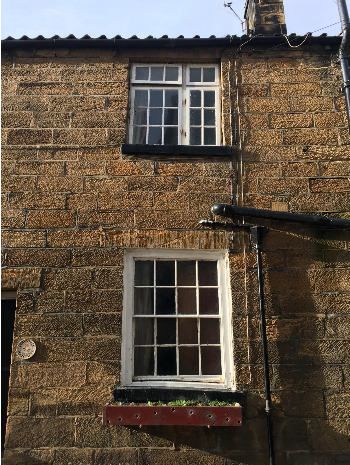
Photograph 6 Part Front Elevation, W2 and W4
