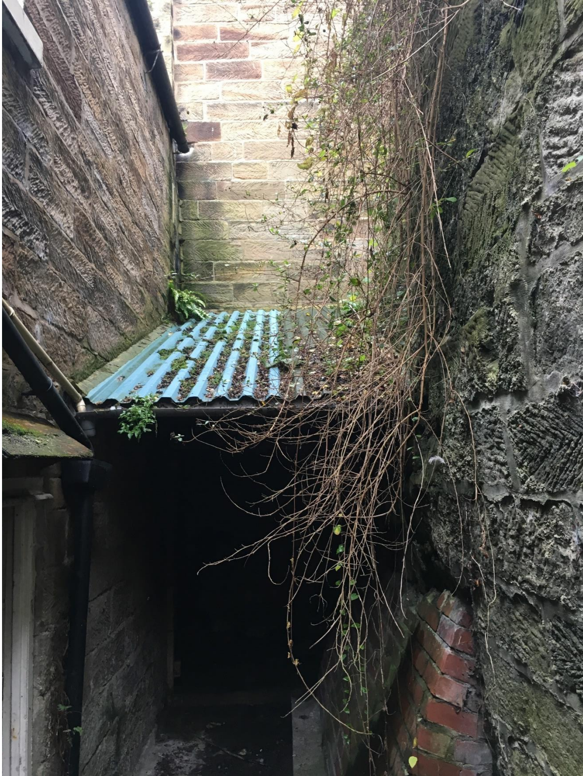
Photograph 9 Rear Yard looking at Party Wall to the south Note; covered area and brick buttress
