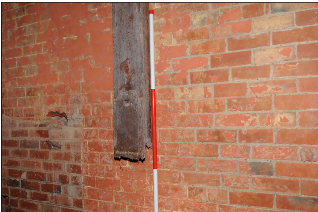
Photograph: 42 Digital Reference: EMBR_060 Description: Detail of the grain Shute on the north wall of the former stable Direction: SE
