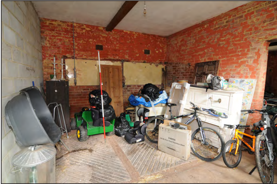
Photograph: 33 Digital Reference: EMBR_051 Description: Former stable area Direction: NE
