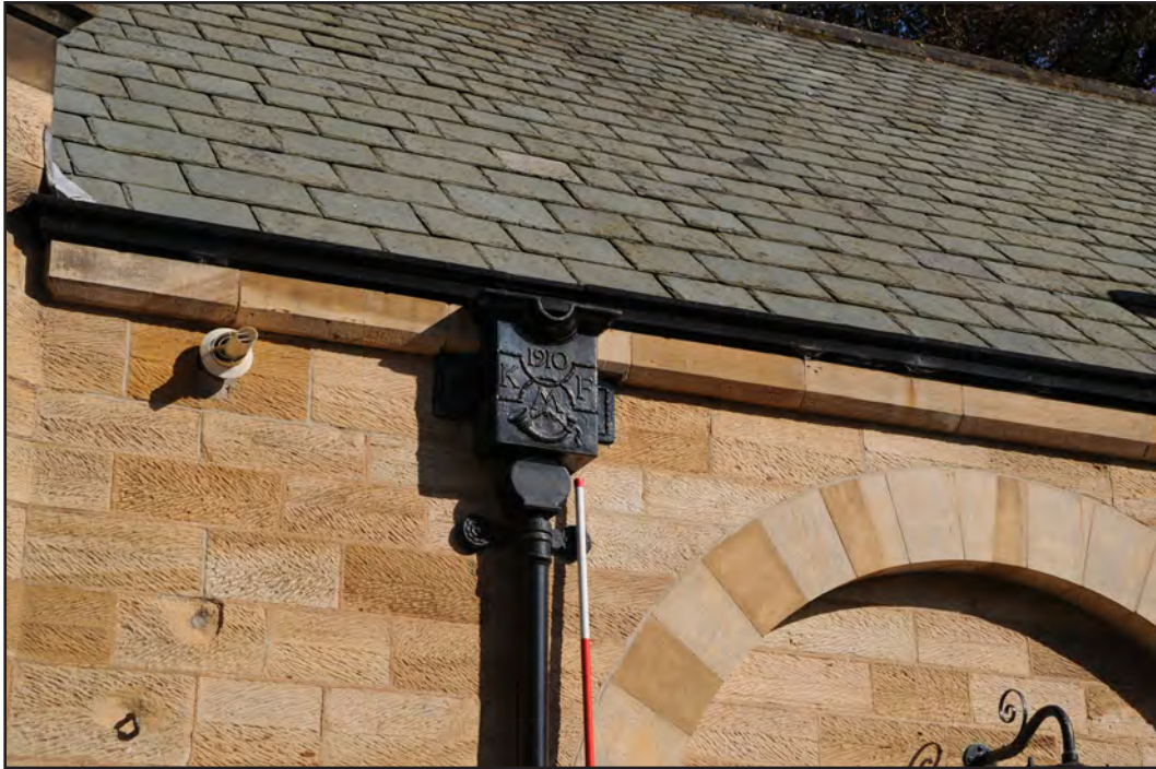
Photograph: 5 Digital Reference: EMBR_016 Description: Dated hopper on the south west wall of the garage Direction: NE
