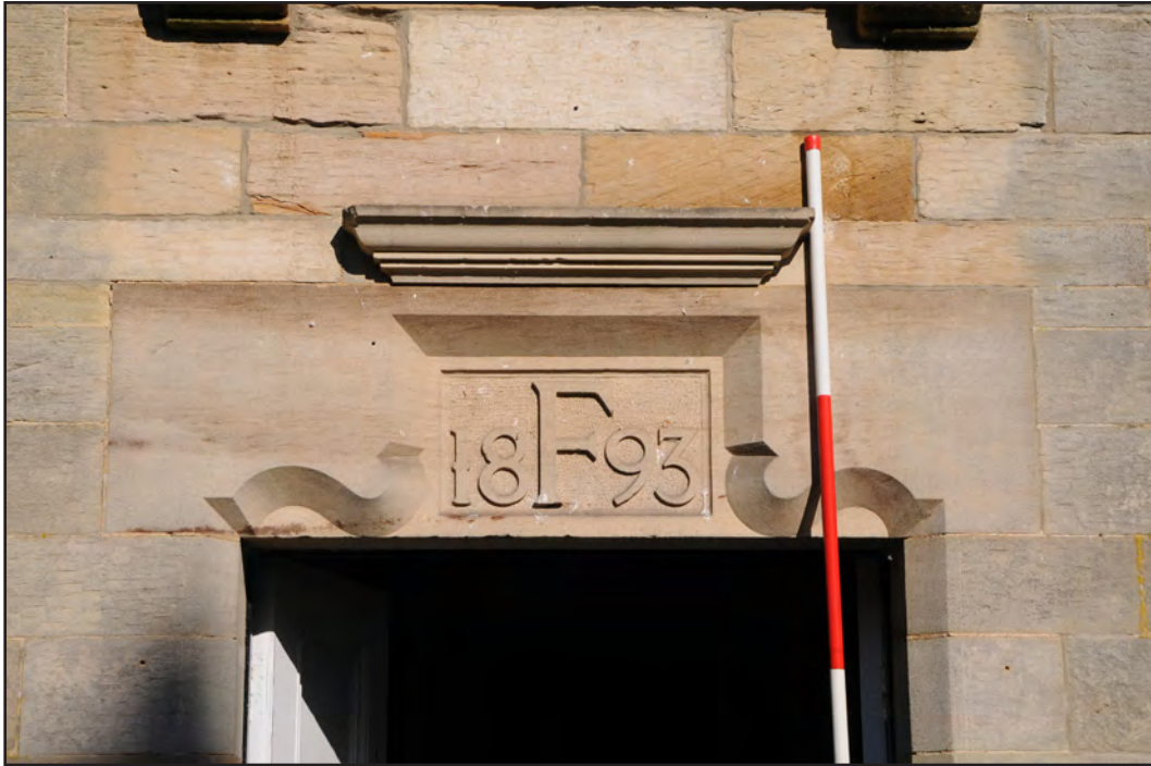
Photograph: 13 Digital Reference: EMBR_017 Description: Carved stone over the doorway to the former stables Direction: N
