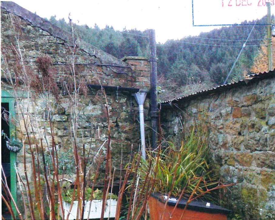
Current Gutter Layout To Rear
