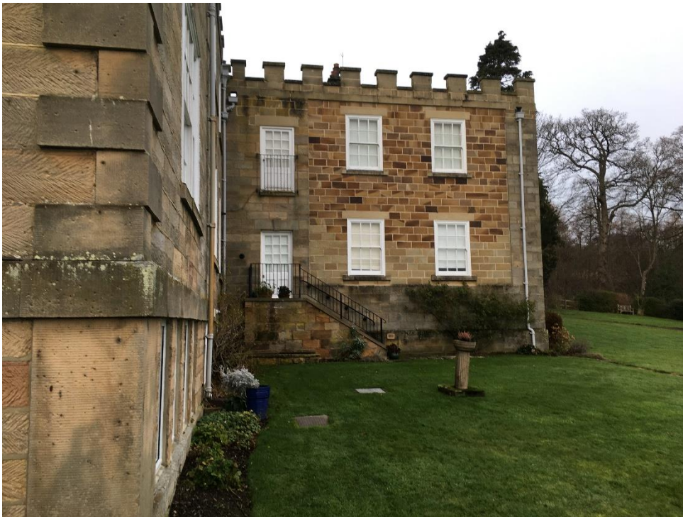
Fig 3. – South elevation of Apartment 11, The Woodlands, Sleights
