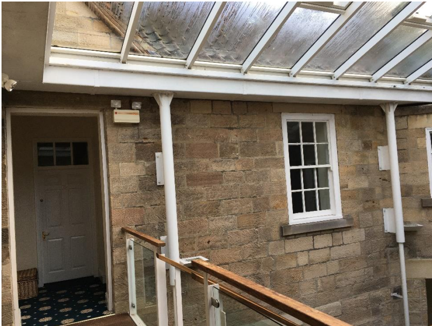
Fig 8. – Main access to first floor passageway and Apartment 11
