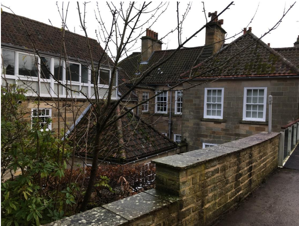
Fig 5. – View from raised walkway looking south east
