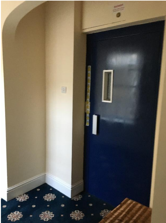
Fig 12. – Former lift entrance door
