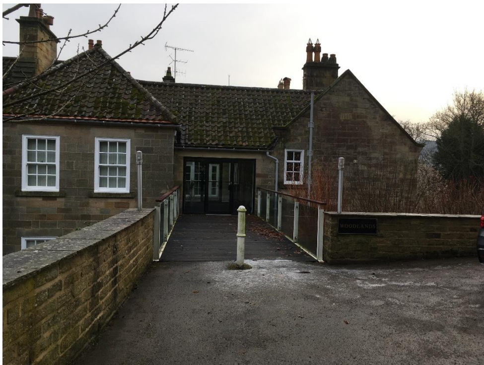
Fig 4. – North elevation accessed by raised walkway
