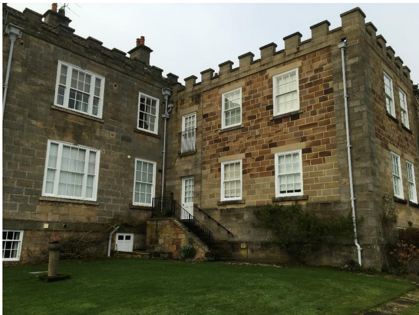
Fig 2. – South elevation of Apartment 11, The Woodlands, Sleights
