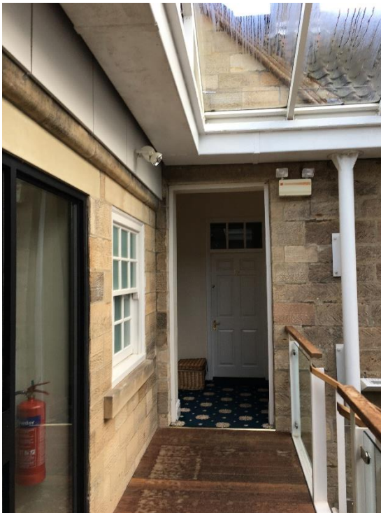
Fig 7. - Access to first floor passageway and Apartment 11
