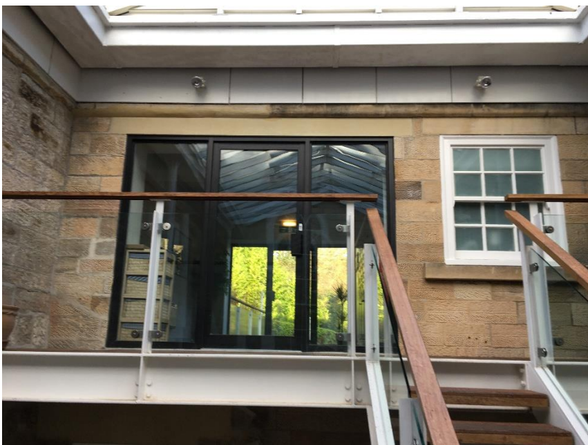
Fig 9. – Looking towards the main entrance
