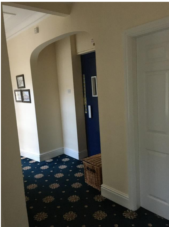
Fig 13. – Entrance to former lift and door to Apartment 11
