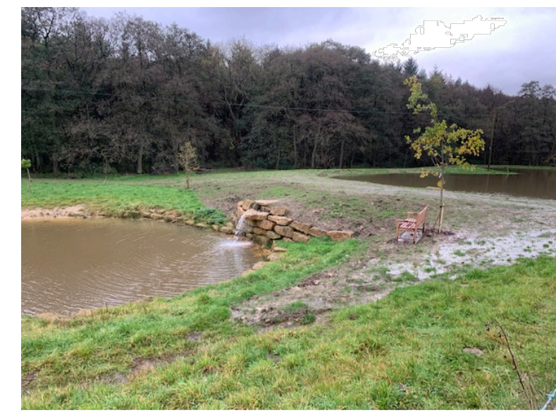
View of outlet to existing pond
