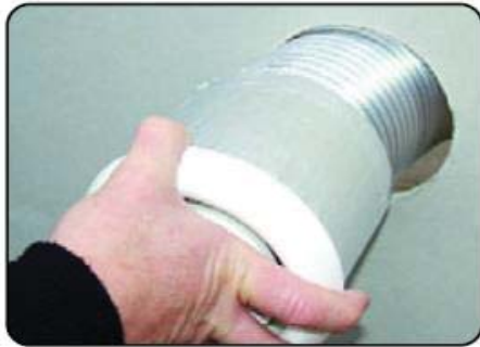
STEP 4: fit the Firoblok sleeve over the vent and fit to the ducting
