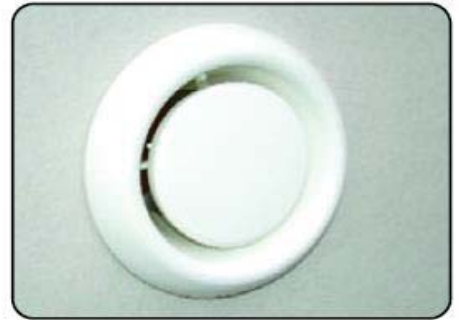
STEP 6: the finished vent with fire protection – a neatly finished job!
