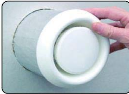
STEP 5: push the assembly back into the substrate until flush
