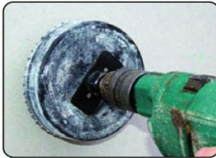
STEP 2: cut out the hole with a powered hole saw or see step 3
