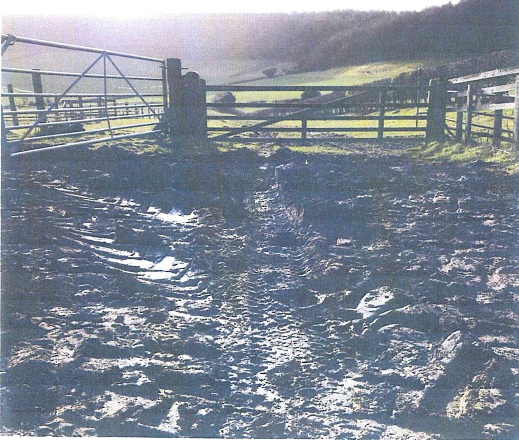
Beacon Brow Road 5 th Feb 2020
